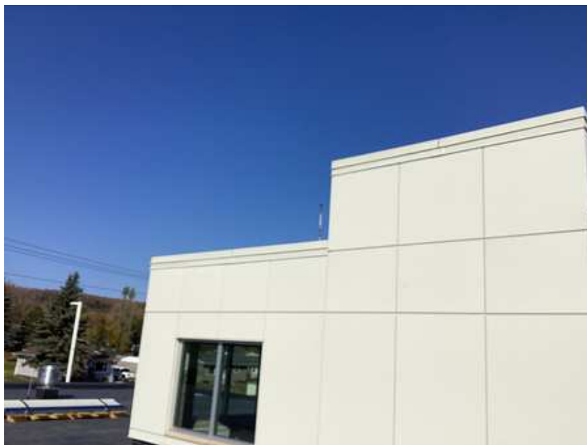
Exterior sheet metal roof coping installed
