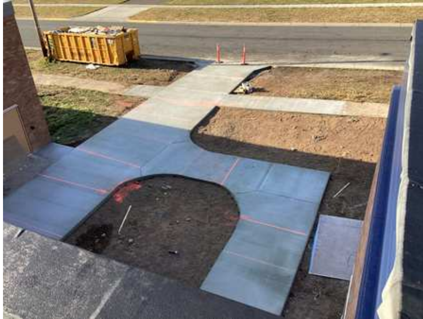
Concrete sidewalks poured
