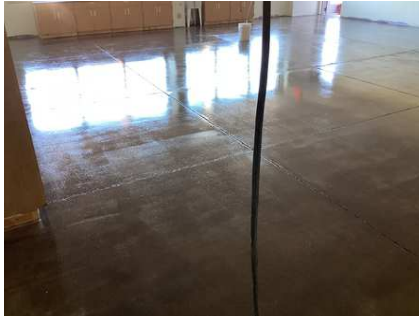
Art Room concrete floor sealed
