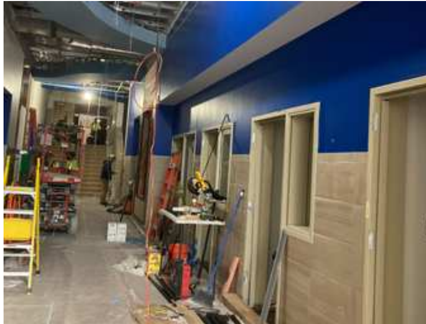
Main corridor, painting, wall tile, flooring and soffits
