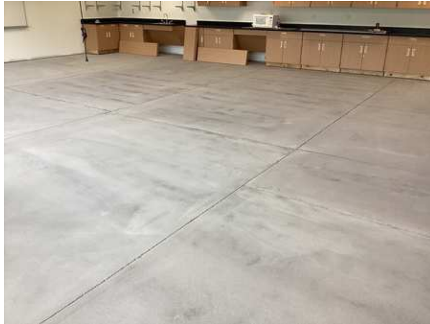
Art Room casework installed and floor preparation for concrete sealing
