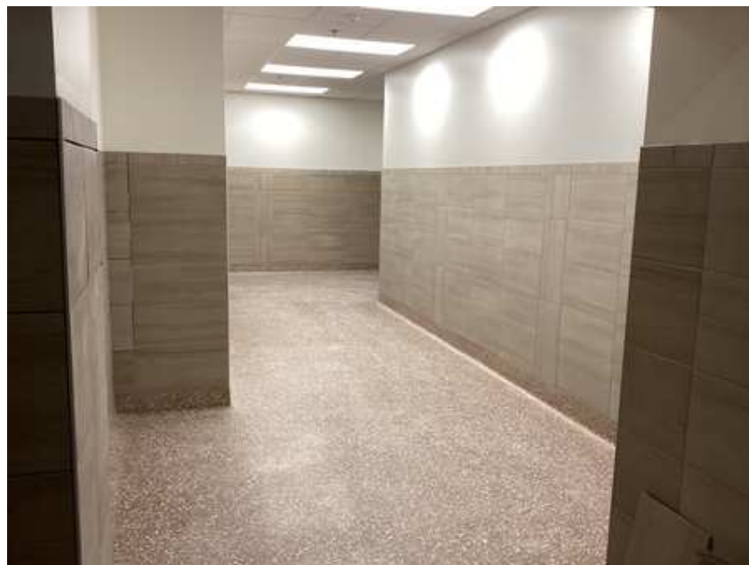
Lower level, corridor/elevator lobby wall tile, flooring and ceiling completed
