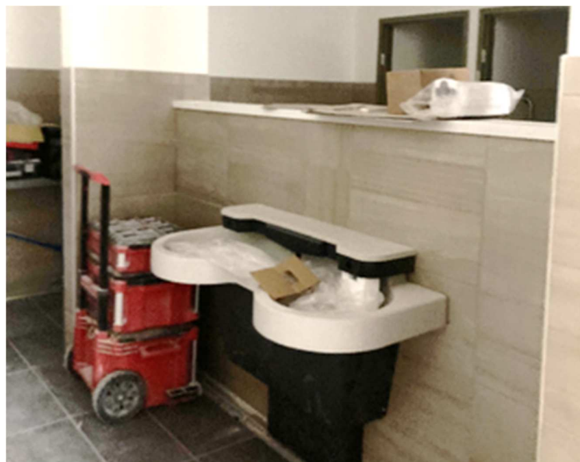
Common area wall tile and lavatory sink
