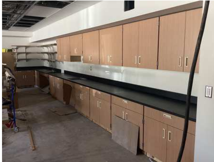
Art Room casework installation
