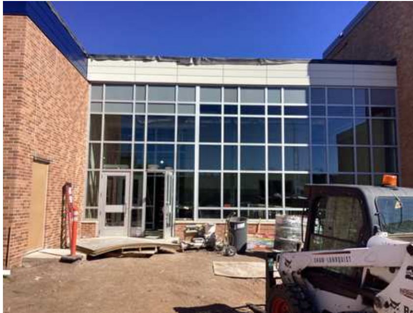
Exterior metal panel installation complete at Music Suite
