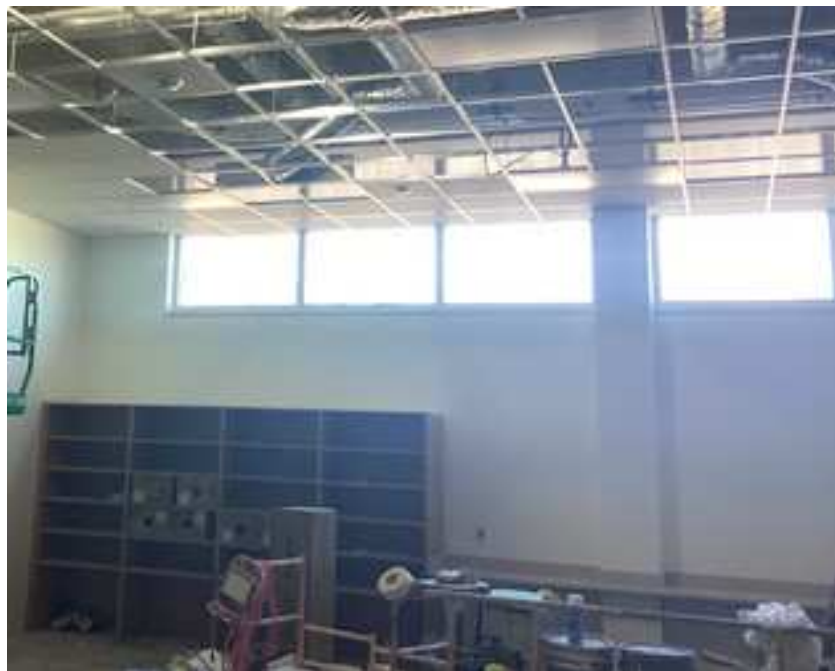
Band Room casework and ceiling grid
