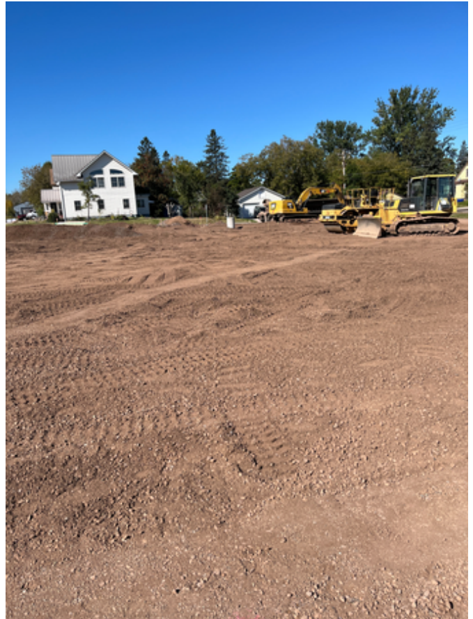
Parking Lot Grading and Curb Preparation.
