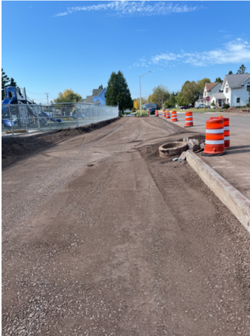
Bus Lane Final Grading
