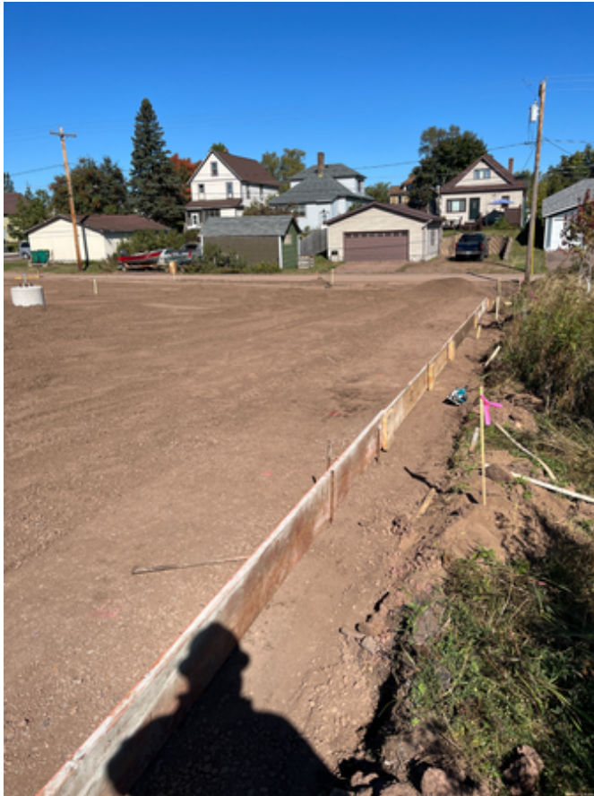
Parking Lot Grading and Curb Preparation.
