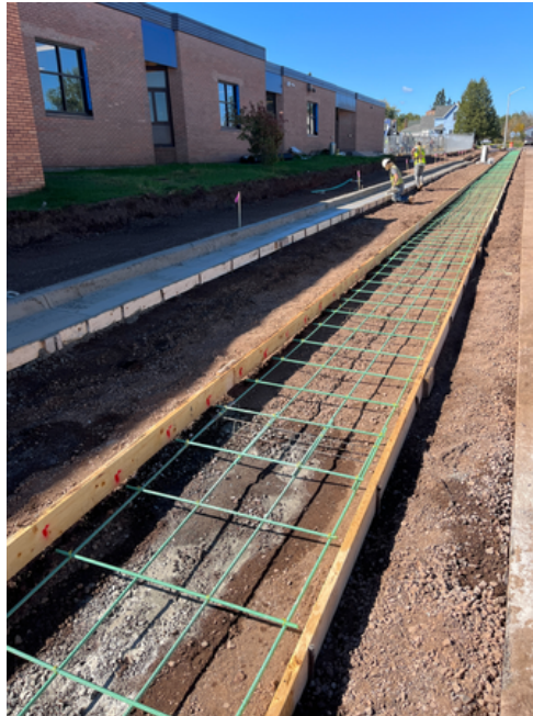
Vally Gutter Form and Rebar
