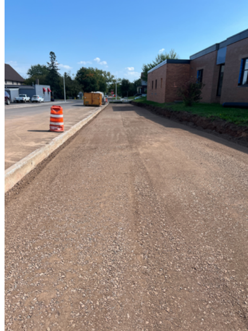
Bus Lane Final Grading
