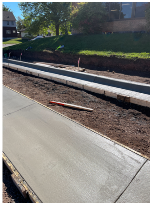
Valley Gutter Poured
