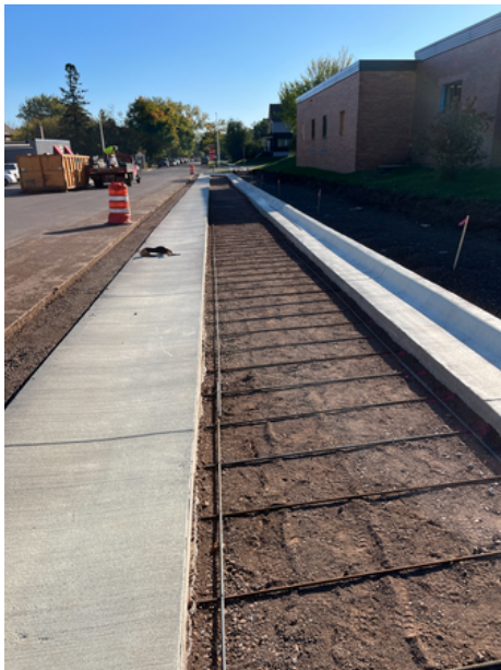
Prepped for Concrete Paving at Bus Lane
