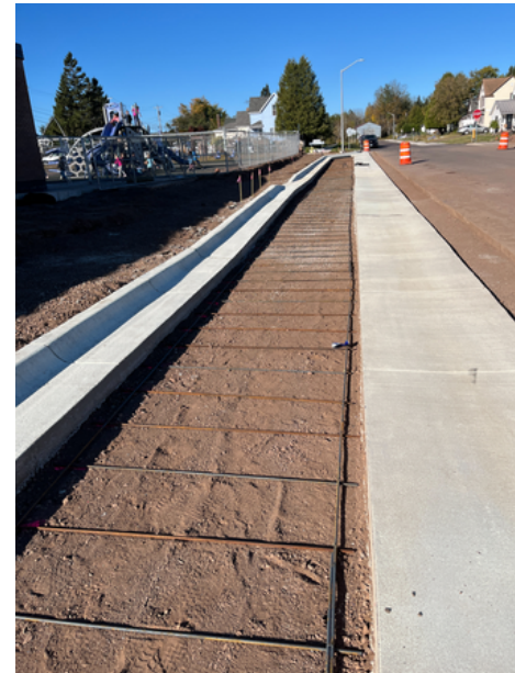
Prepped for Concrete Paving at Bus Lane
