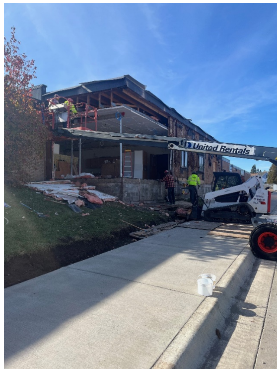
Area B Exterior Wall Demolition/Replacement
