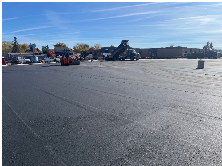
Parking lot Paving
