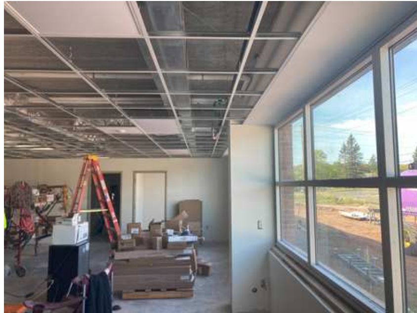
Art Room ceilings and light fixtures
