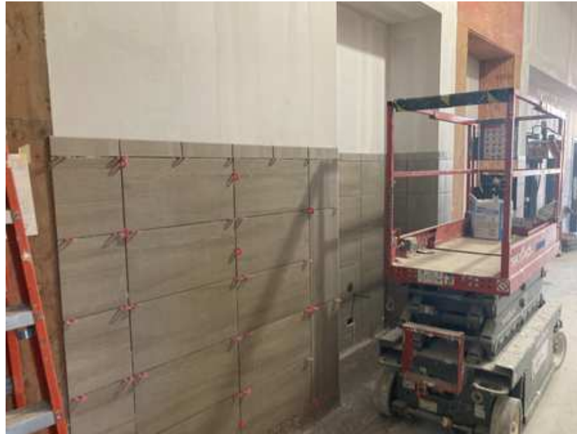
Corridor wall tile installation in Music Suite
