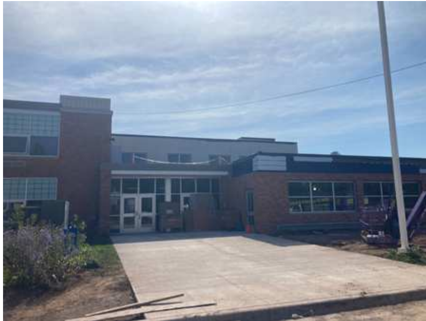
Exterior metal panel installation at Music Suite
