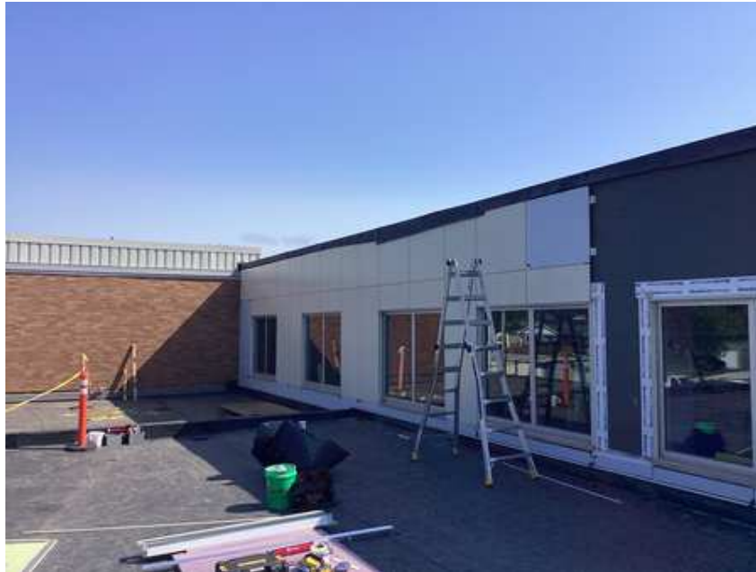
Exterior metal panel installation at Music Suite
