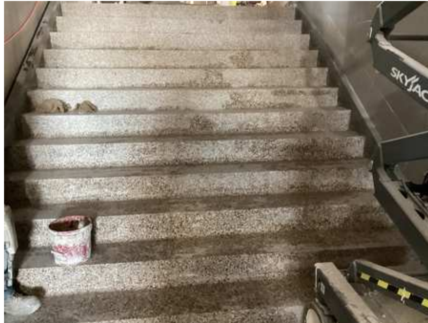
Terrazzo stair poured in Music Suite
