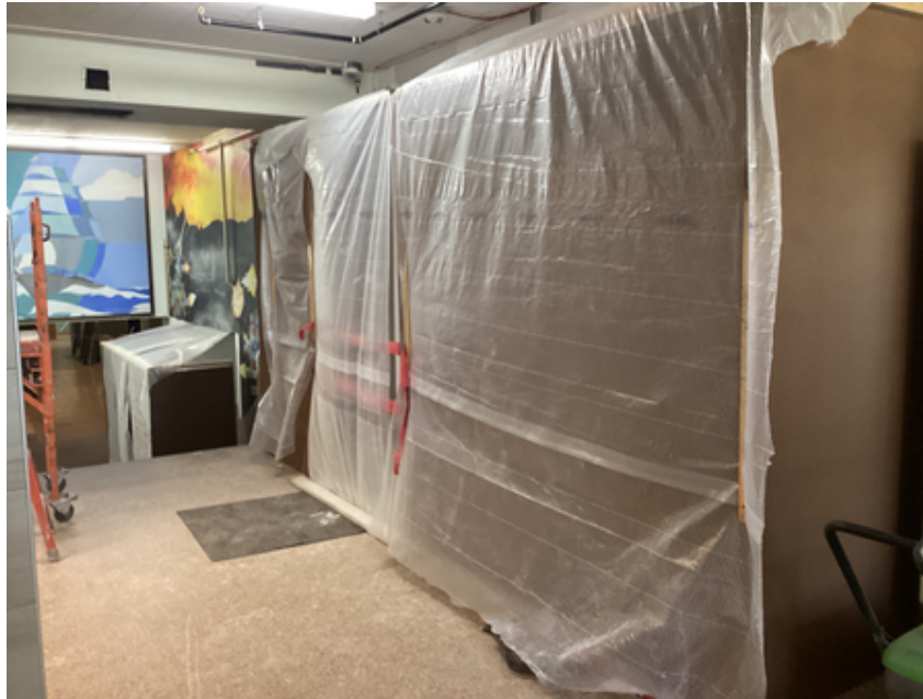
Temporary construction wall
