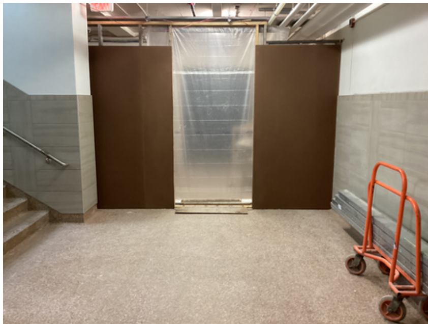
Temporary construction wall
