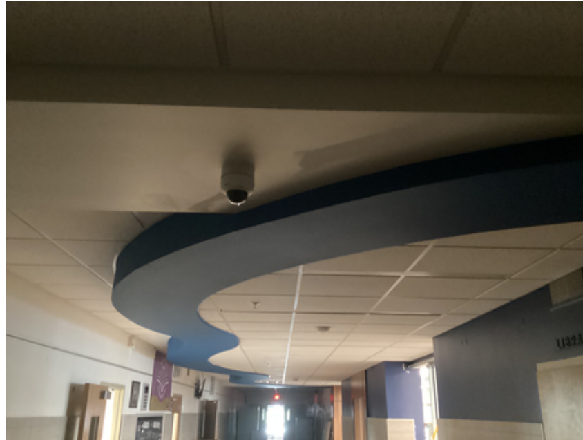
Corridor soffits completed
