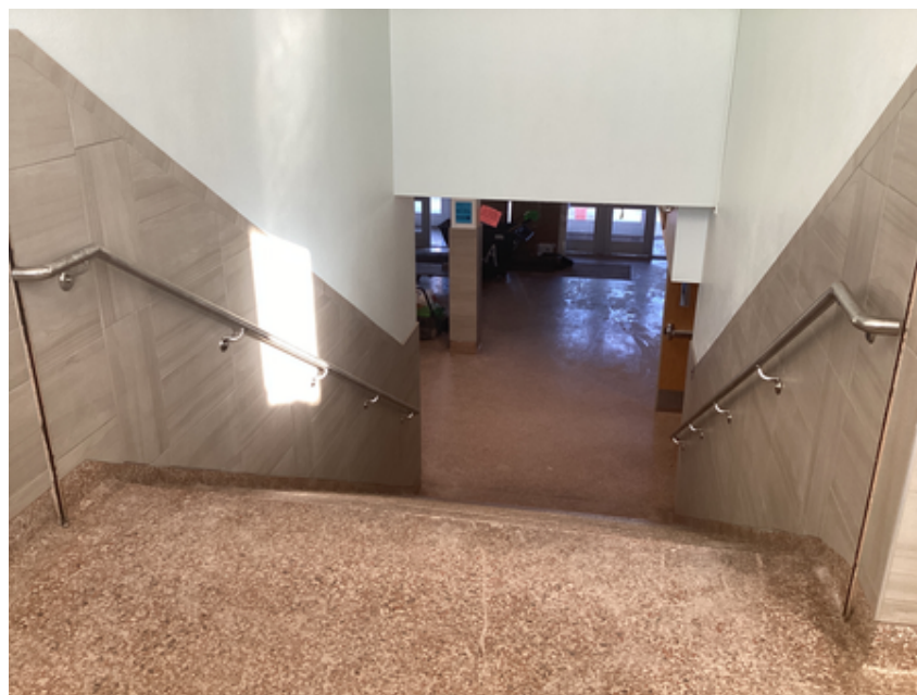
Stairwell wall tile and hand rails completed
