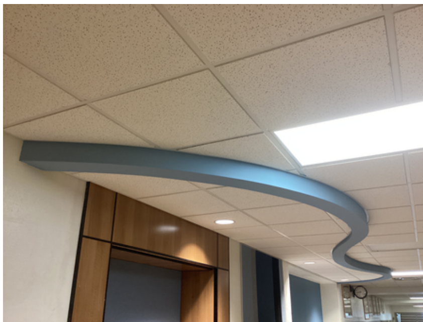
Corridor nooks/displays completed
