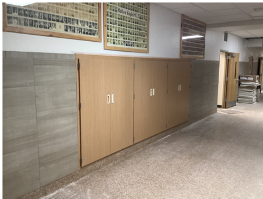
Corridor wall tile and cabinetry
