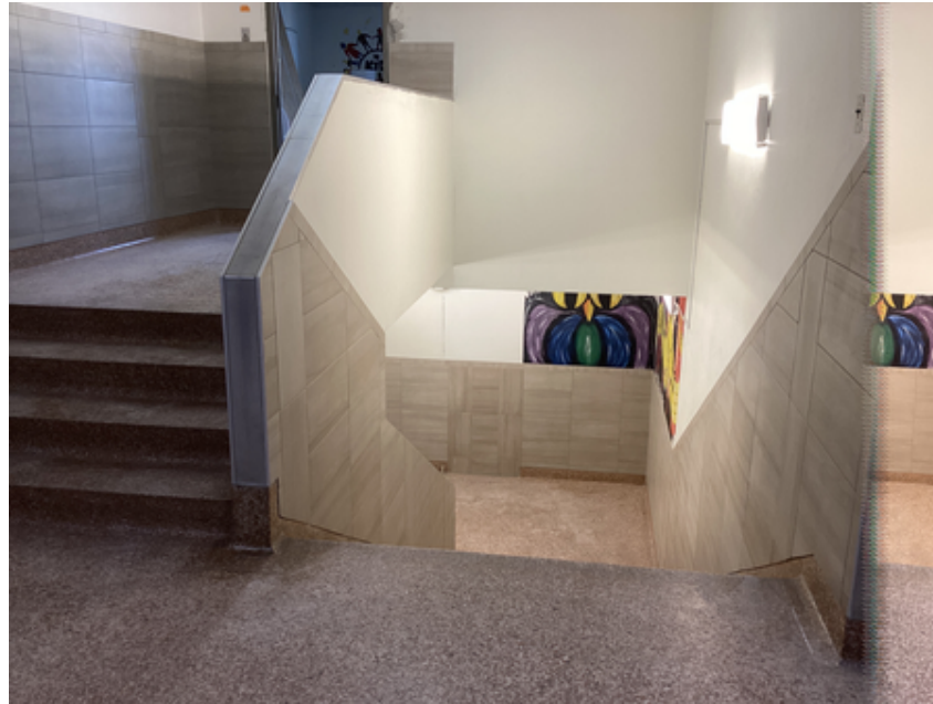
Stairwells wall tiled
