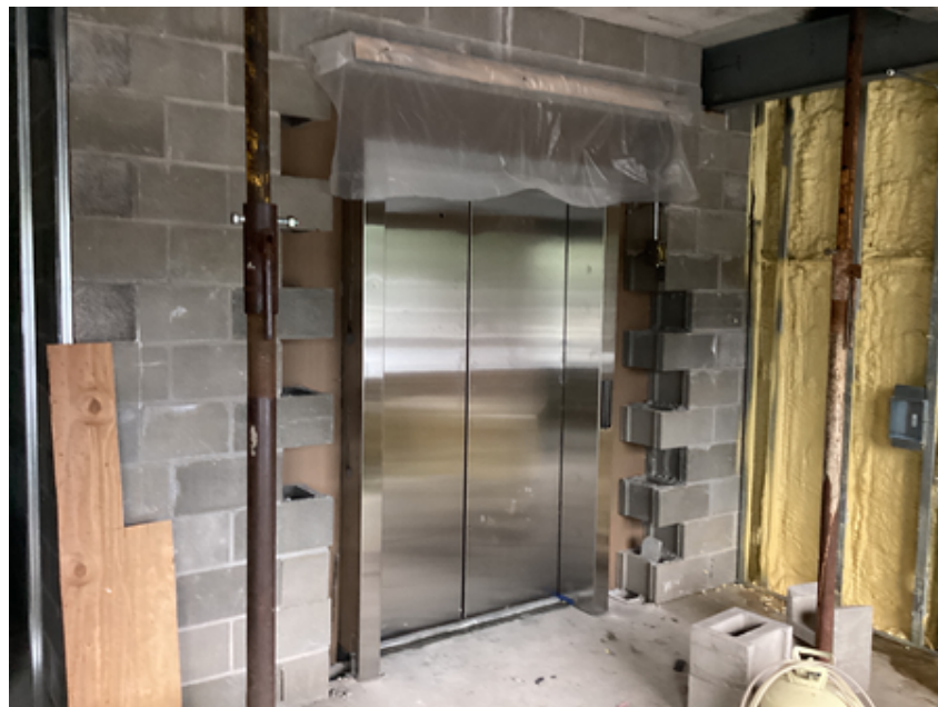
Elevator Install at Music Suite
