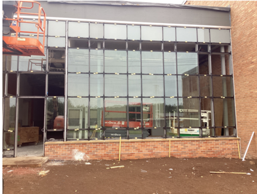
Glazing installed at Music Exterior Curtain Wall
