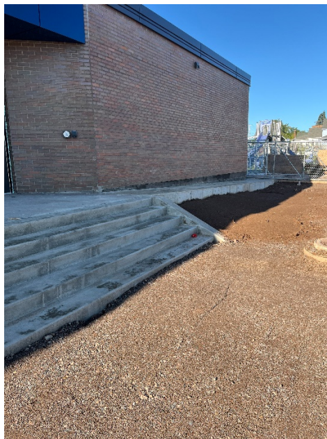
New North Stairs and ADA Ramp
