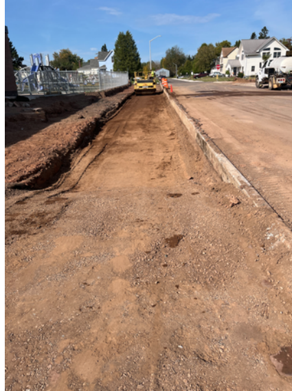
Bus Lane Excavation and preparation of Concrete work.
