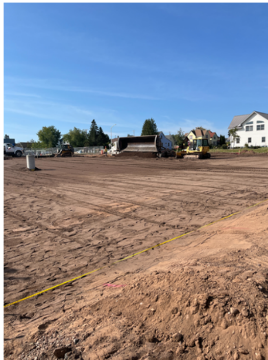
Parking Lot Base installation. Light Pole Bases installed.
