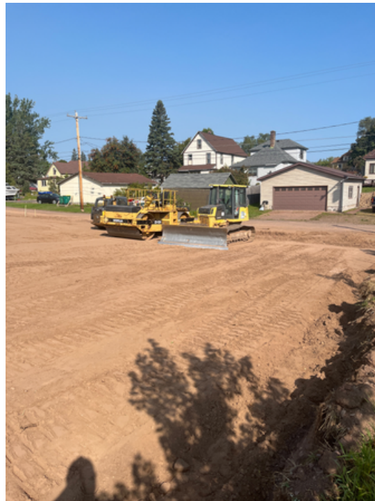
Parking Lot Light Pole Bases Installed. Sand Sub-base in place.
