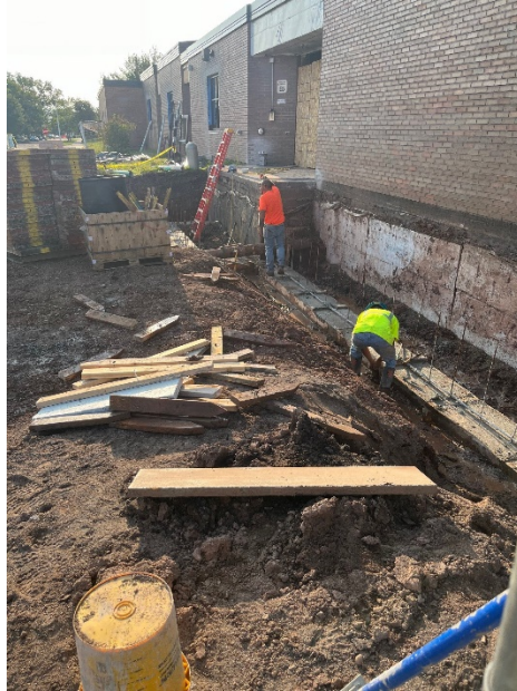
ADA Ramp and Steps at North side of Building.
