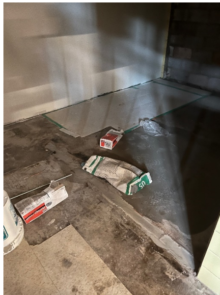
Floor Prep and VCT Patching
