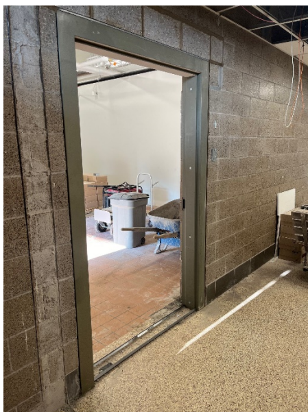
Final Door Frame installations.
