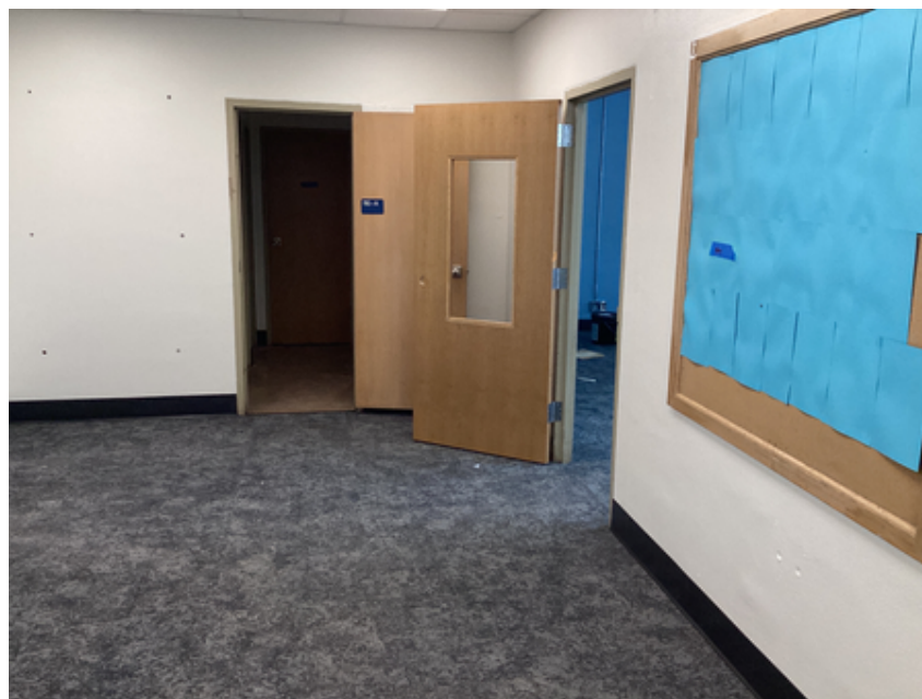
Flooring complete in old Admin areas/Tech offices
