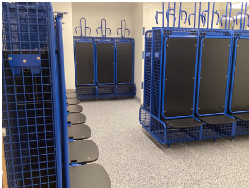
Locker installation in boys' locker room
