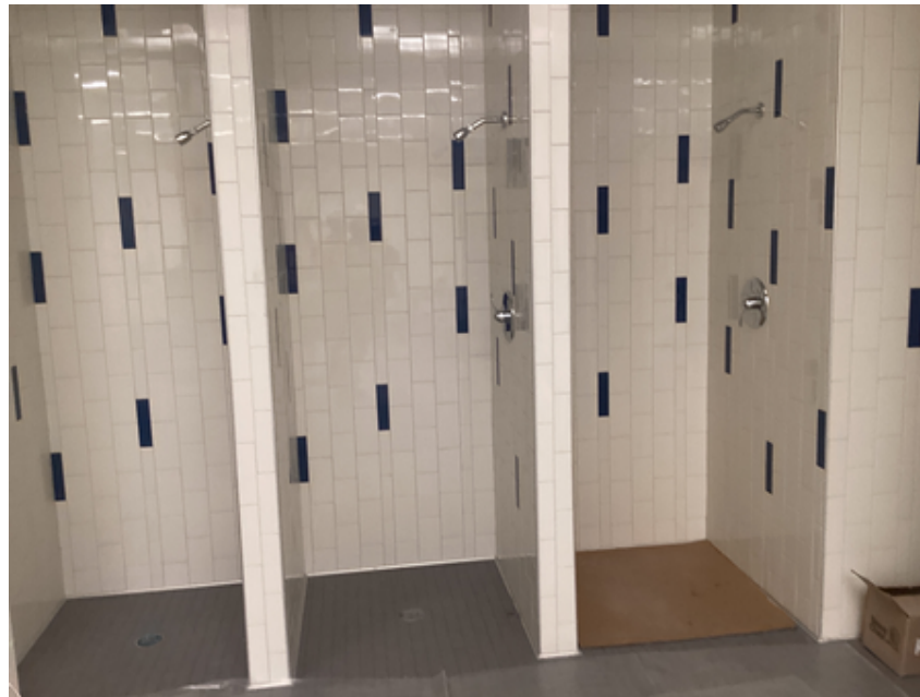
Girls locker room wall and floor tile complete
