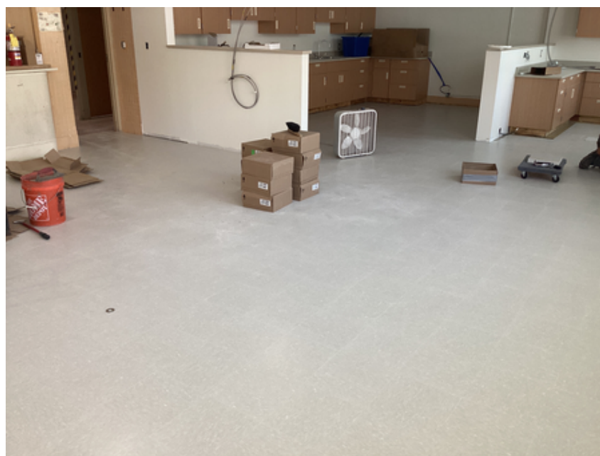
Casework and flooring installation in FACS
