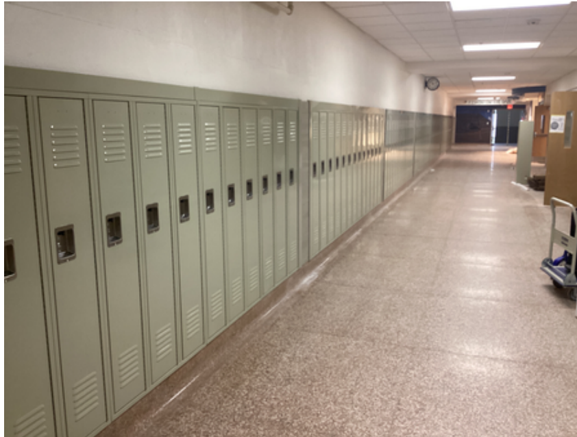
Corridor locker installation
