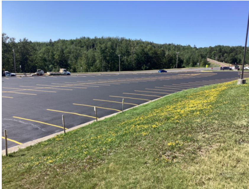
Parking lot crack sealed, recoated, and painted
