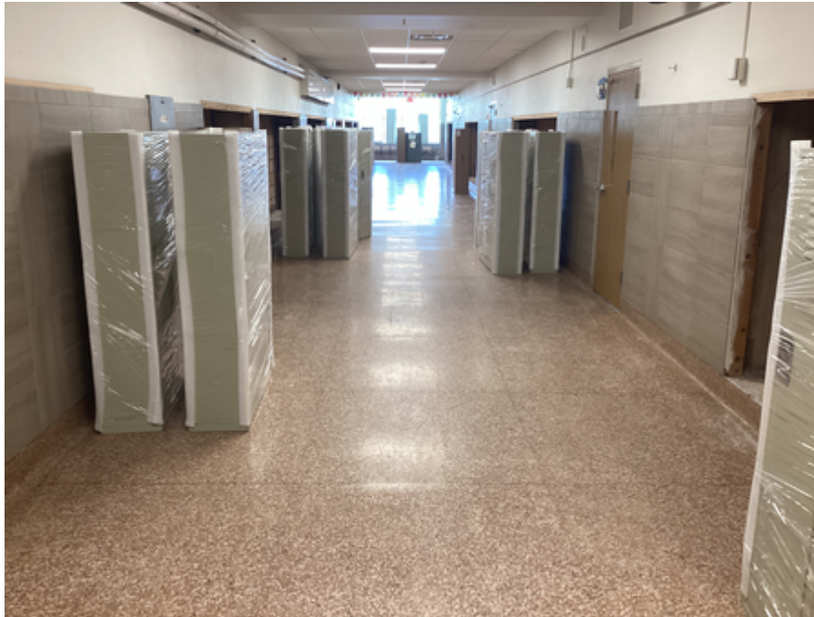
Corridor lockers delivered and staged ready for install
