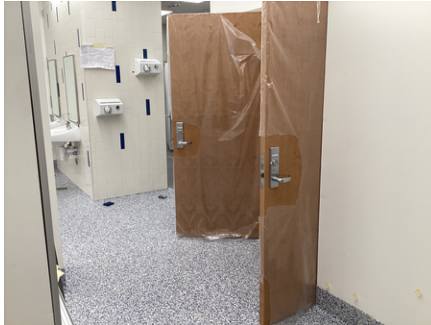
Doors and hardware installation boys' locker room
