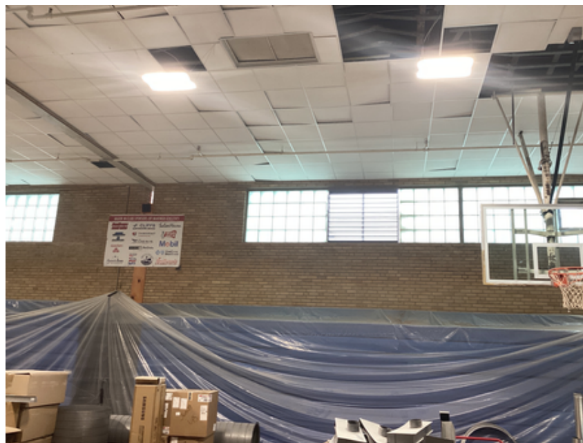
Competition gym lights installed
