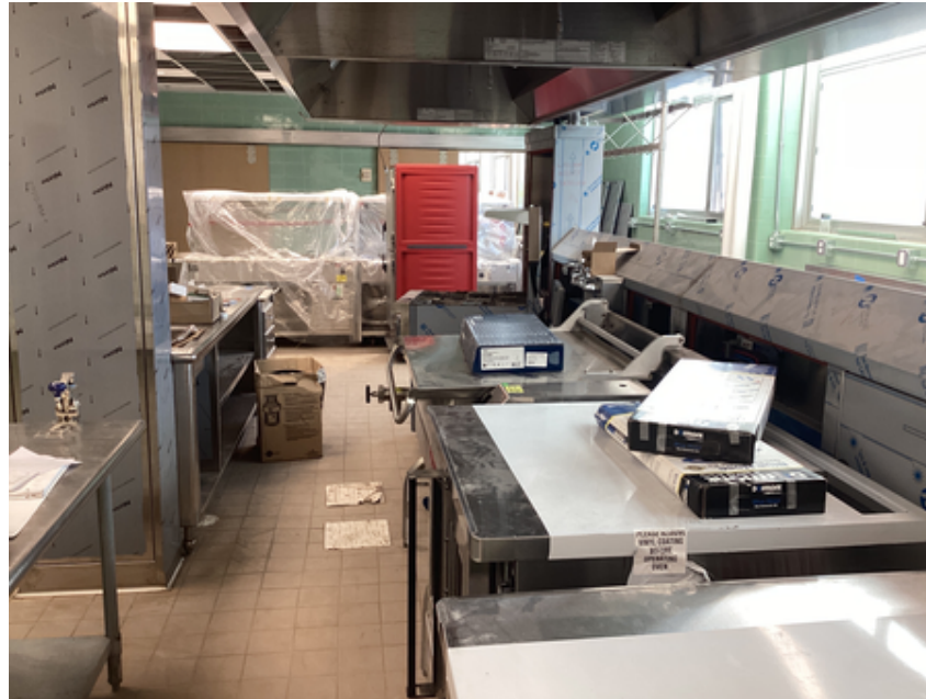
Stainless and food service equipment installation in kitchen
