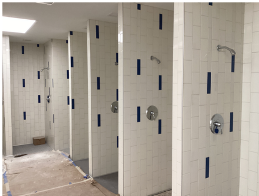
Wall and floor tile installation in girls' locker room
