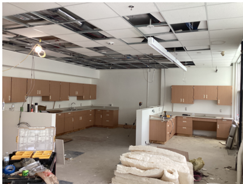
FACS casework installation
