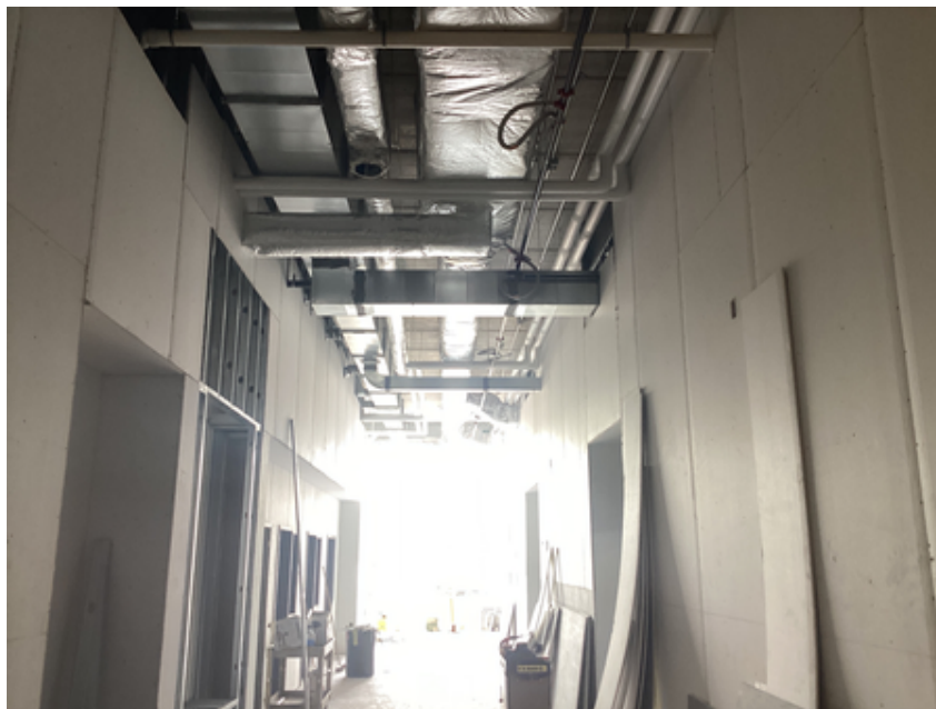
Stairwell wall framing in Music Addition
