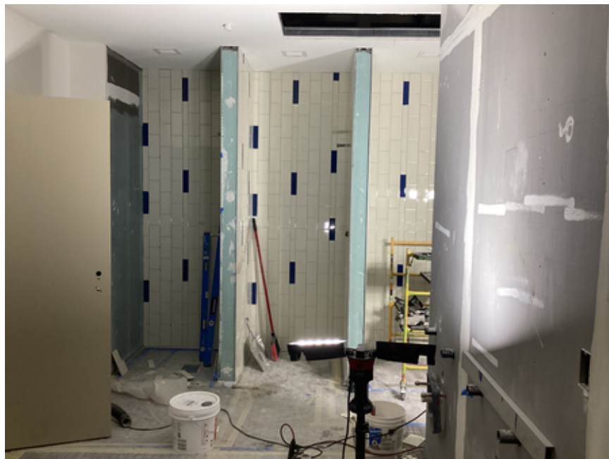
Wall tile installation in girls' locker room
