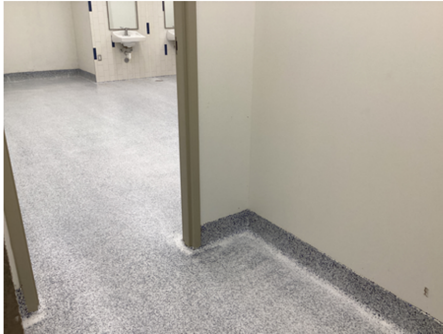
Epoxy flooring in boys' locker room
