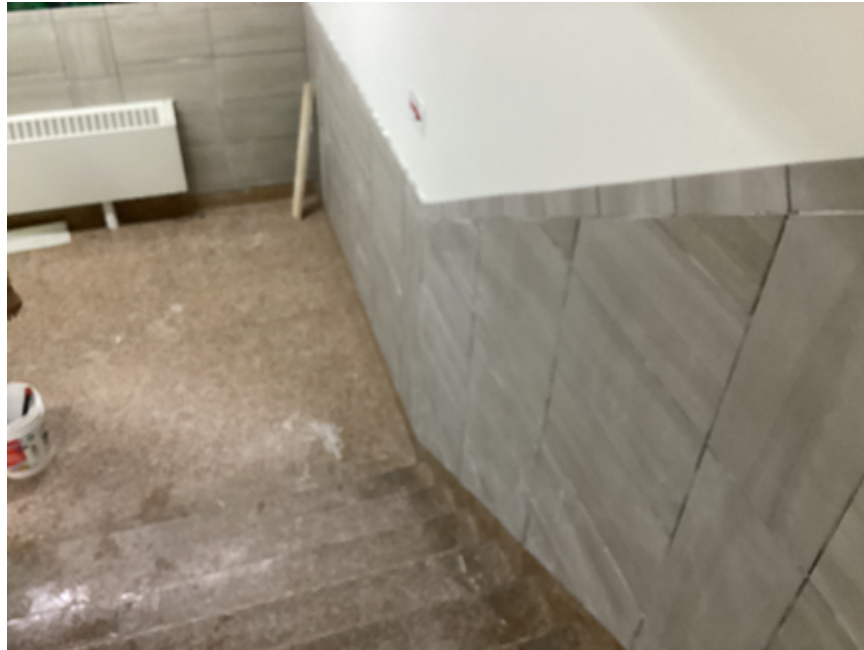
Wall tile in stairwells
