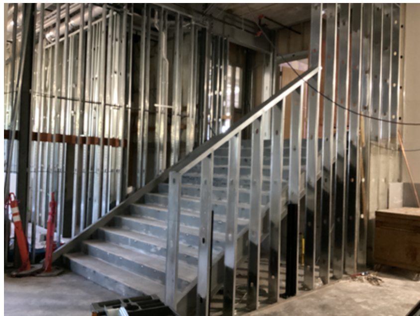
Stairwell wall framing in Music Addition
