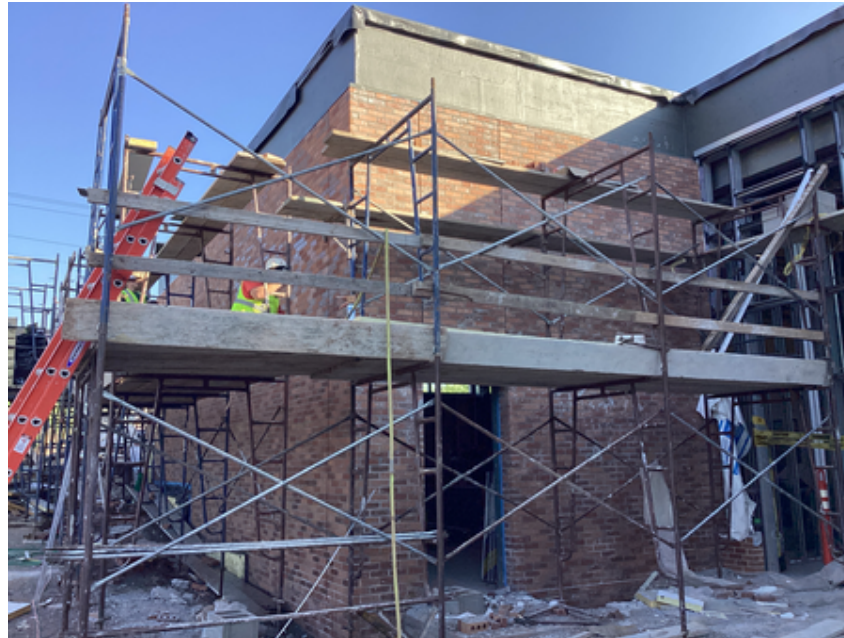
Last portion of brickwork Area B Music Suite
