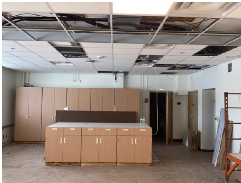
Casework installation in old administrative area
