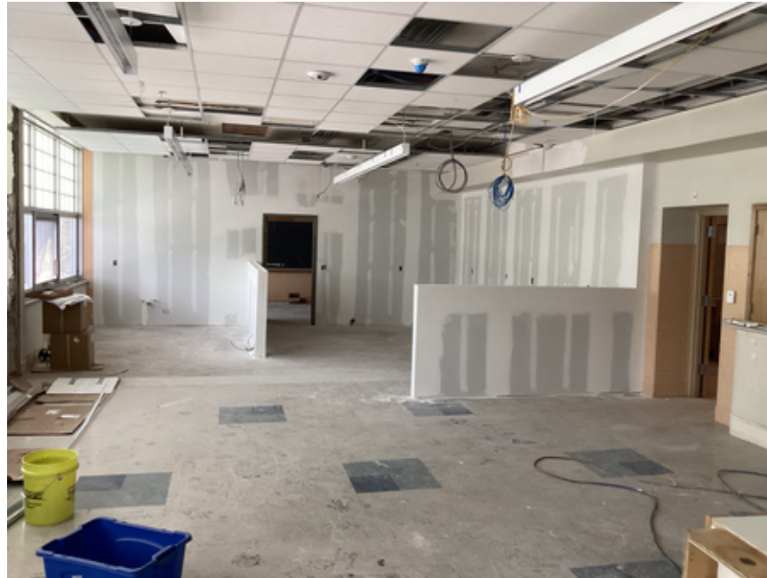
FACS Lab drywall work
