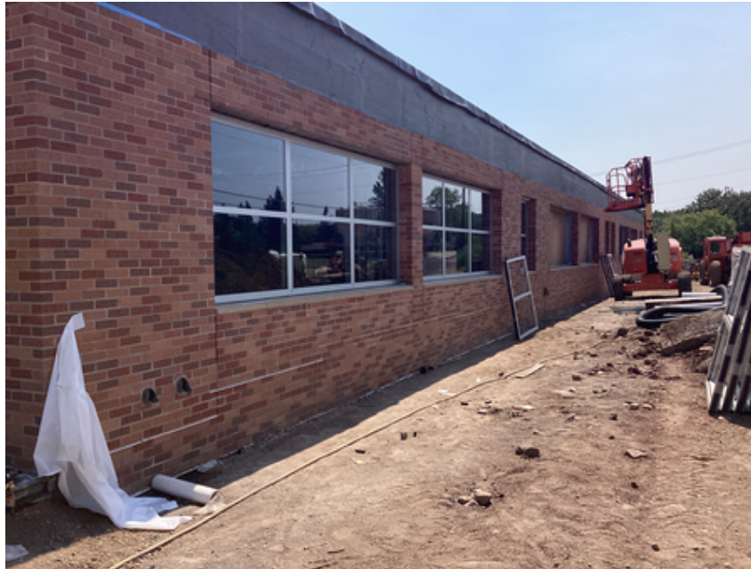
Brickwork Area B Music Suite
