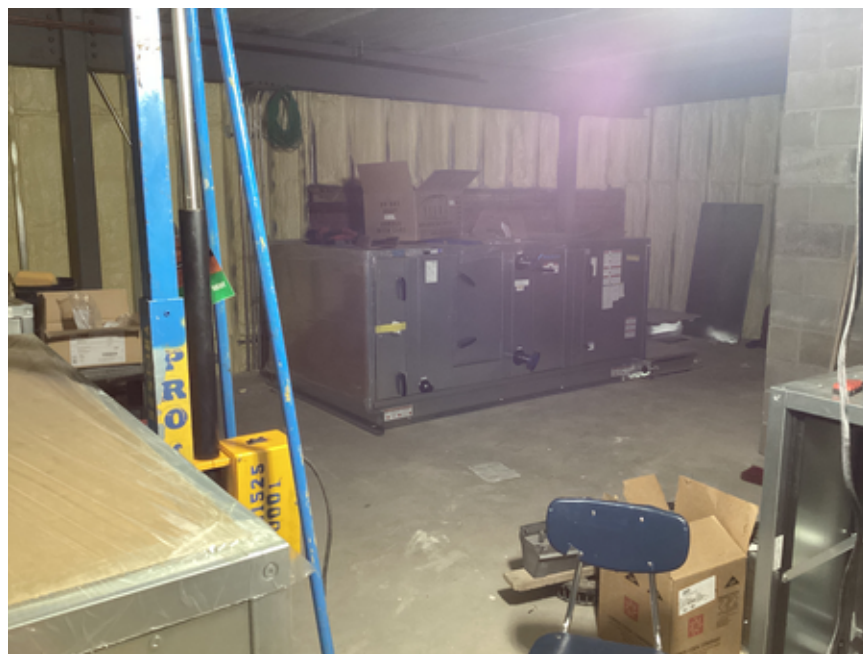
Air handling units being set
