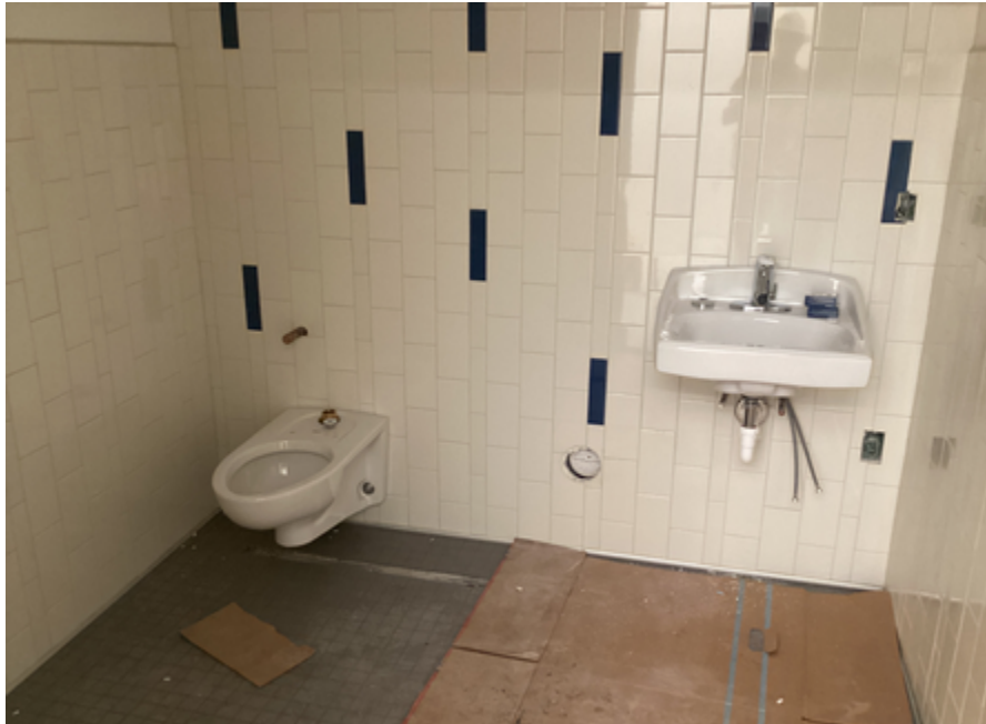
Plumbing fixtures installation in boys locker room
