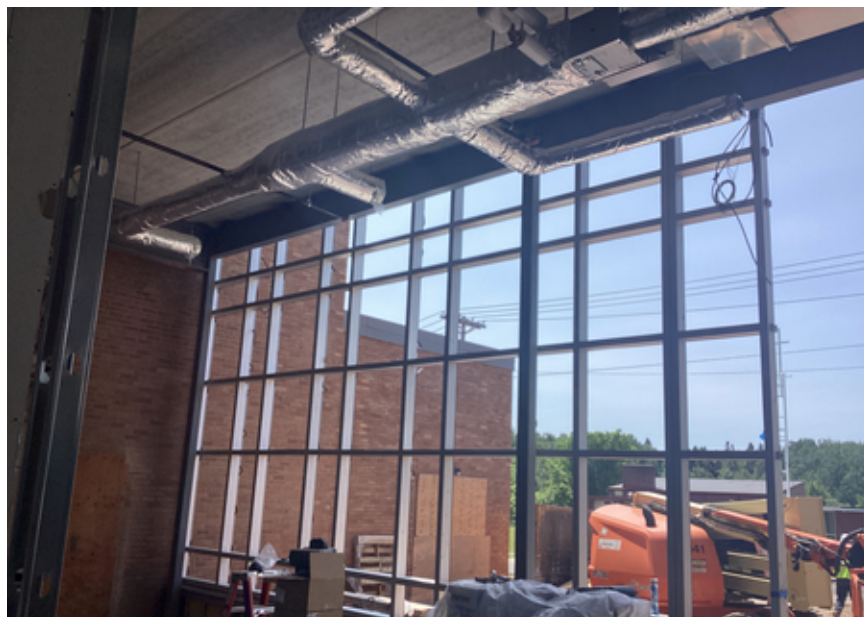
Curtain wall, aluminum storefront framing in Area B Music Suite
