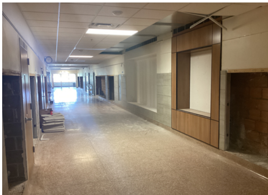
Corridor tile work and seating nook framing
