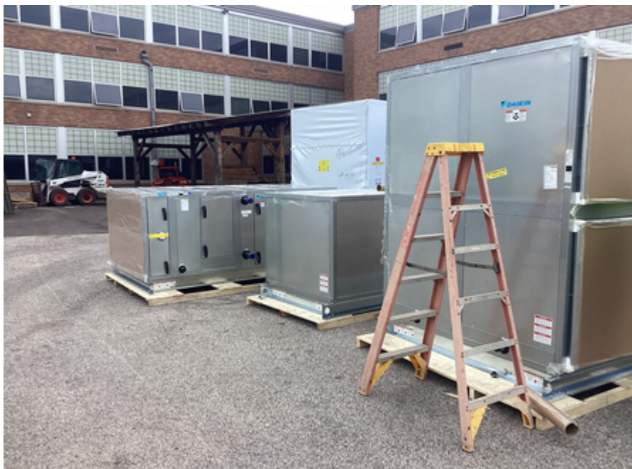
Air handling units delivered
