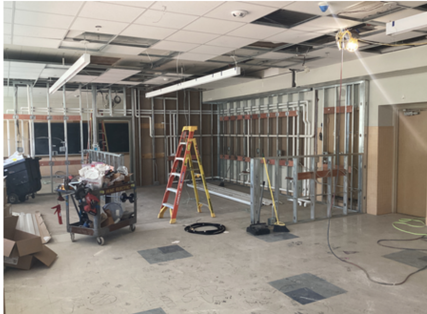
FACS Lab mechanical and electrical rough ins
