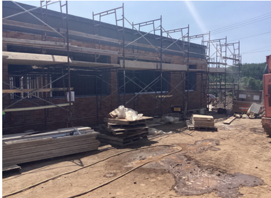
Brickwork Area B Music Suite
