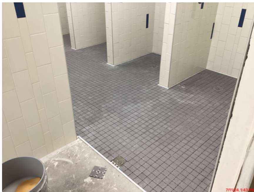
Boys locker room wall and floor tile
