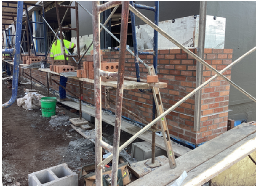
Brickwork Area B Music Suite
