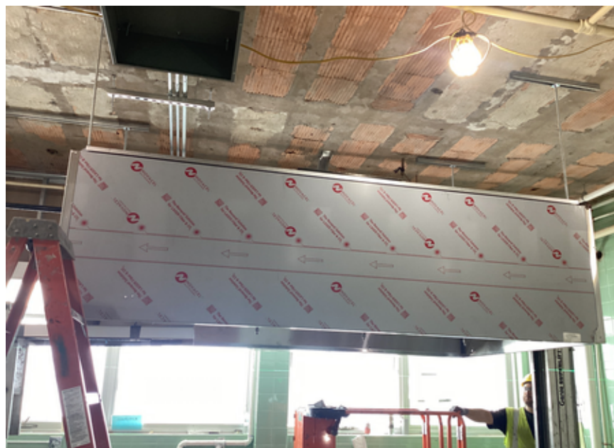
Kitchen hood installation
