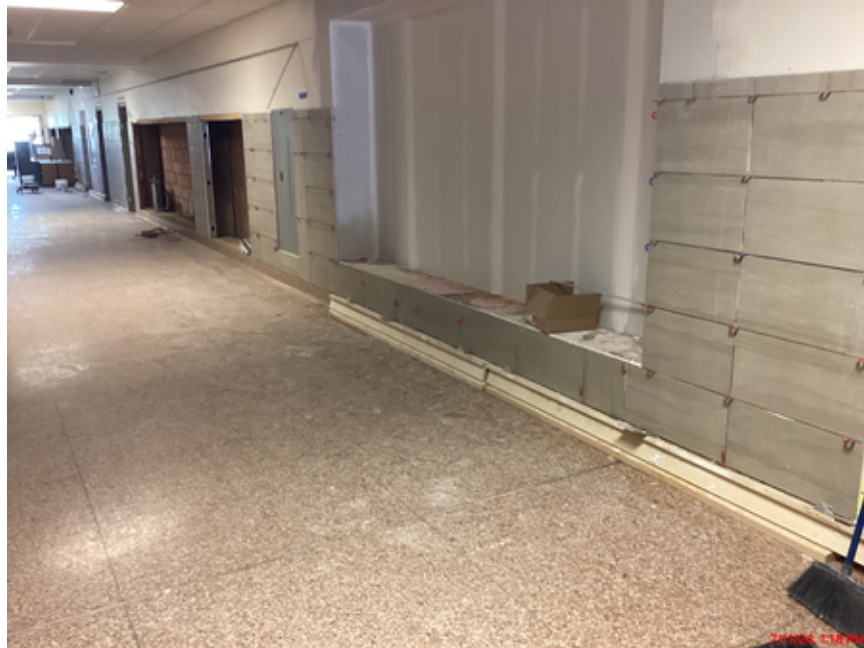
Corridor tile work and seating nook framing
