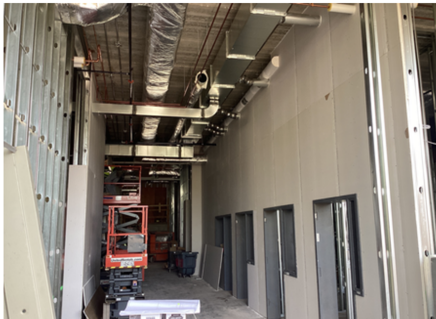
Drywall framing Area B Music Suite
