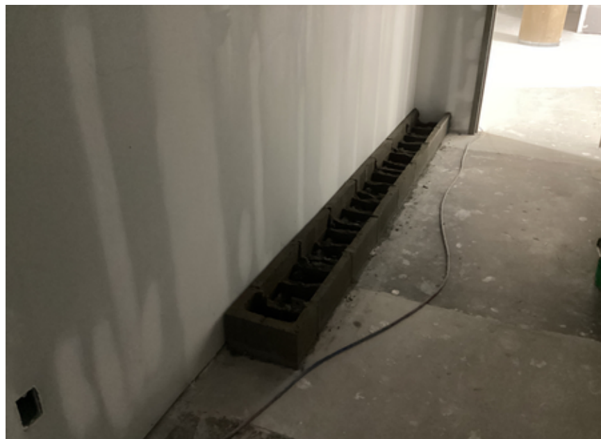
Girls locker room locker bases
