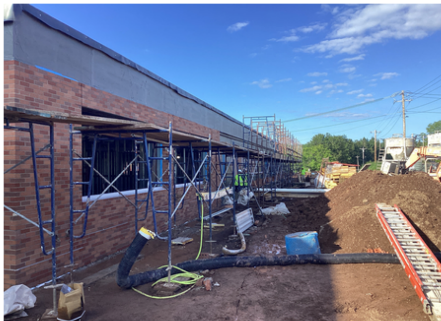
Brickwork Area B Music Suite
