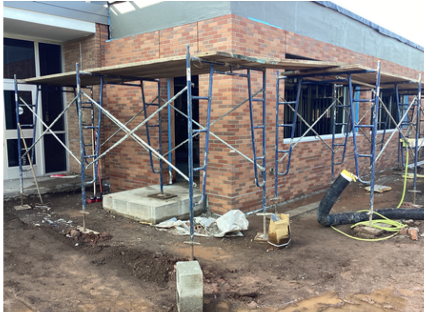
Brickwork Area B Music Suite
