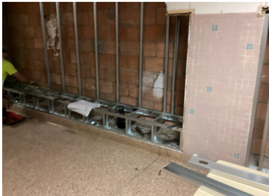
Corridor locker bases framing
