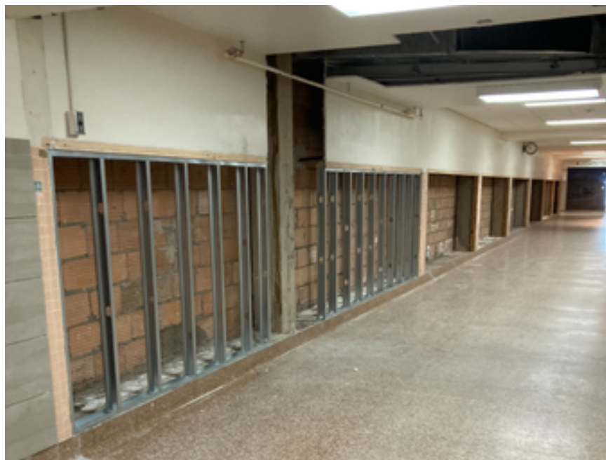
Corridor wall framing
