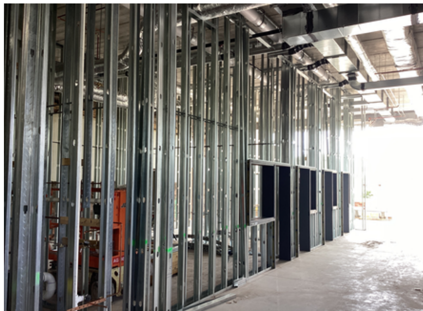
Wall framing, and mechanical/electrical rough in Area B Music Suite
