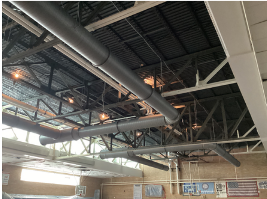
Gym ductwork installation
