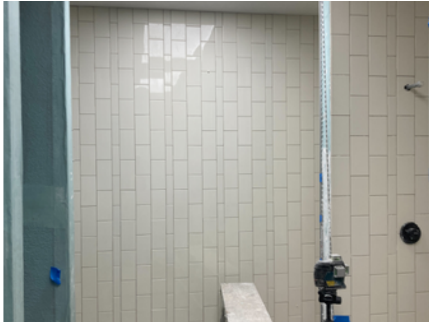
Boys locker room wall tile
