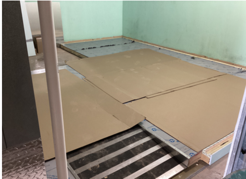
Freezer modifications for Kitchen
