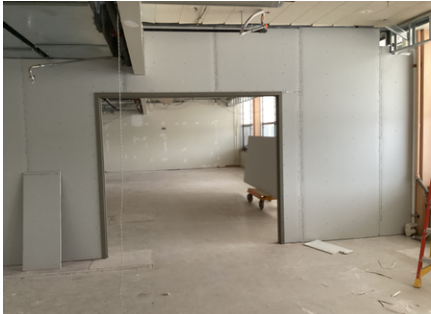
New FACS drywall
