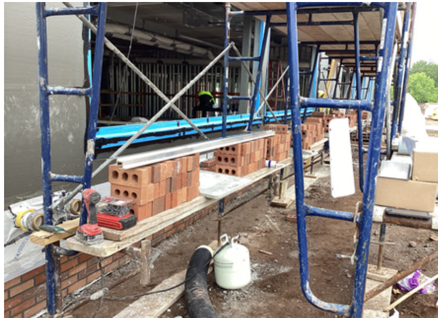
Brickwork Area B Music Suite
