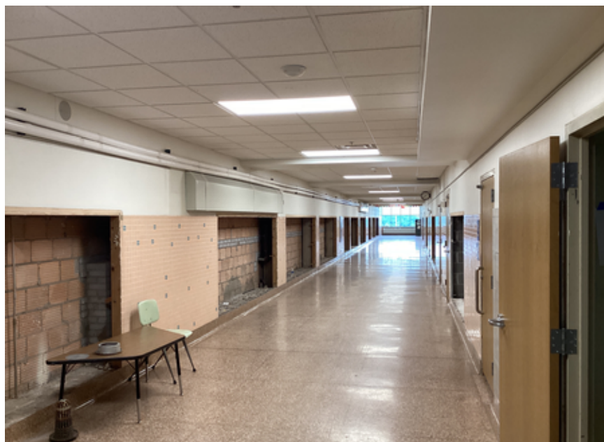
Lockers removed in corridors
