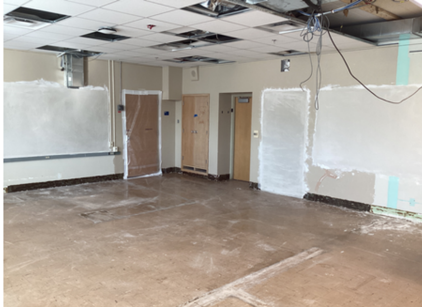
Old Admin/new Tech wall patchwork
