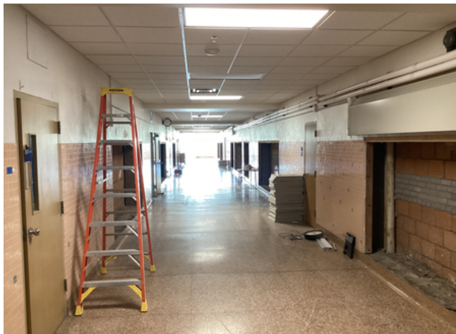
All lockers removed
