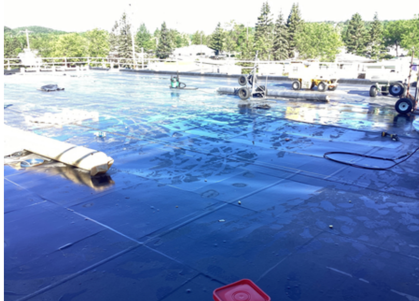
Roofing for Area B Music Suite
