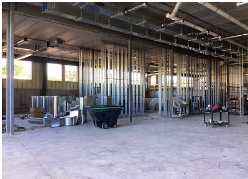
Wall framing, and mechanical/electrical rough in Area B Music Suite
