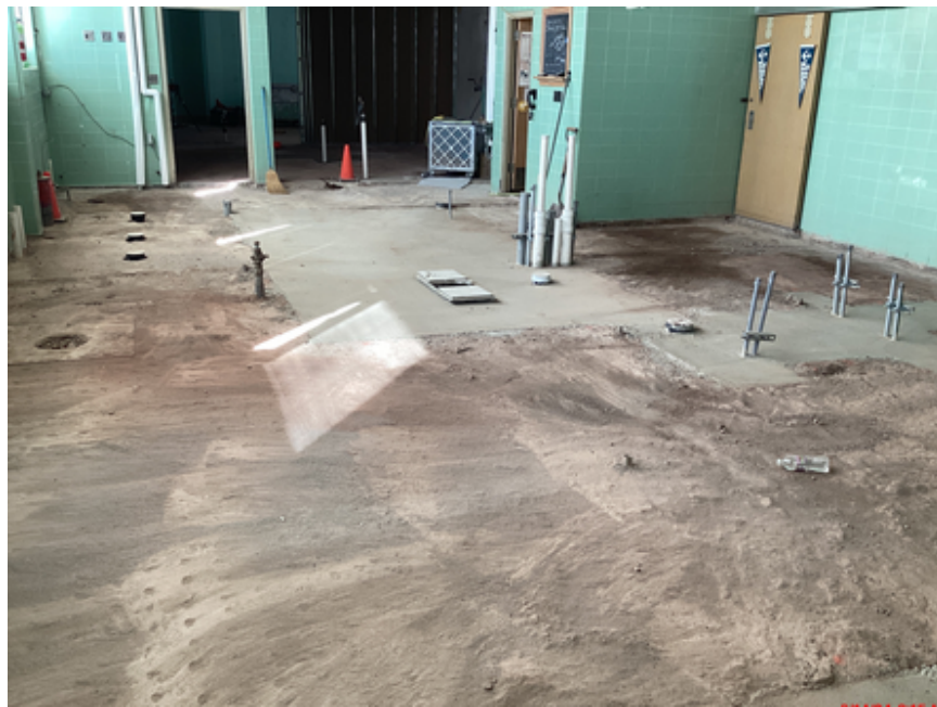
Kitchen floor poured back
