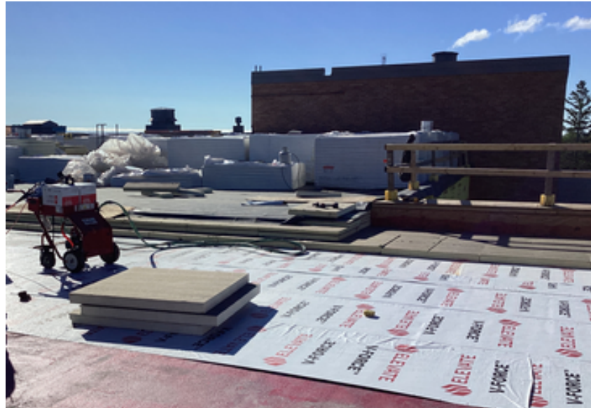
Roofing for Area B Music Suite
