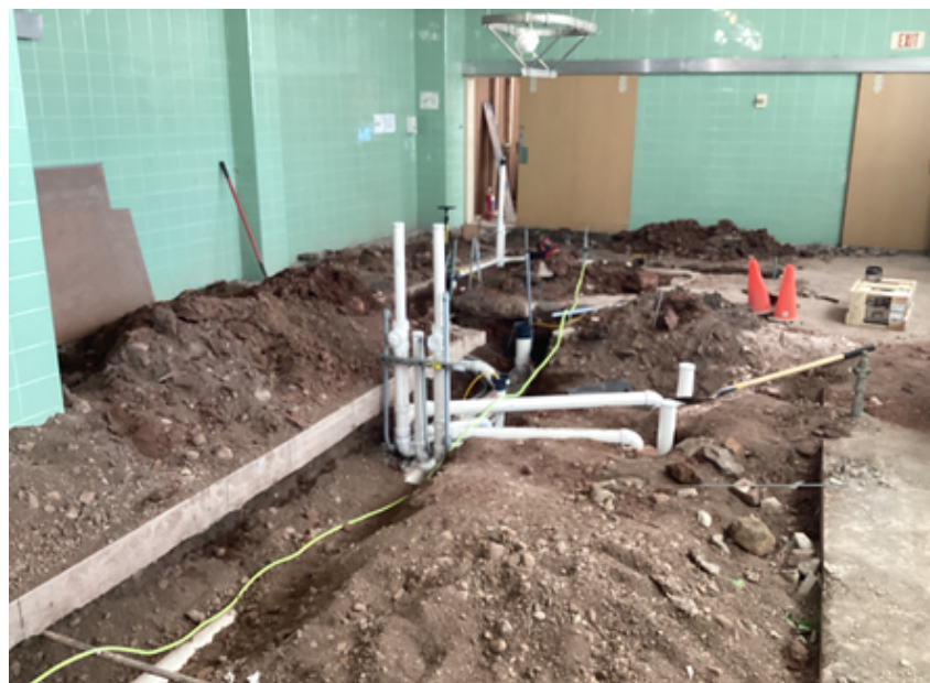
Kitchen mechanical rough in
