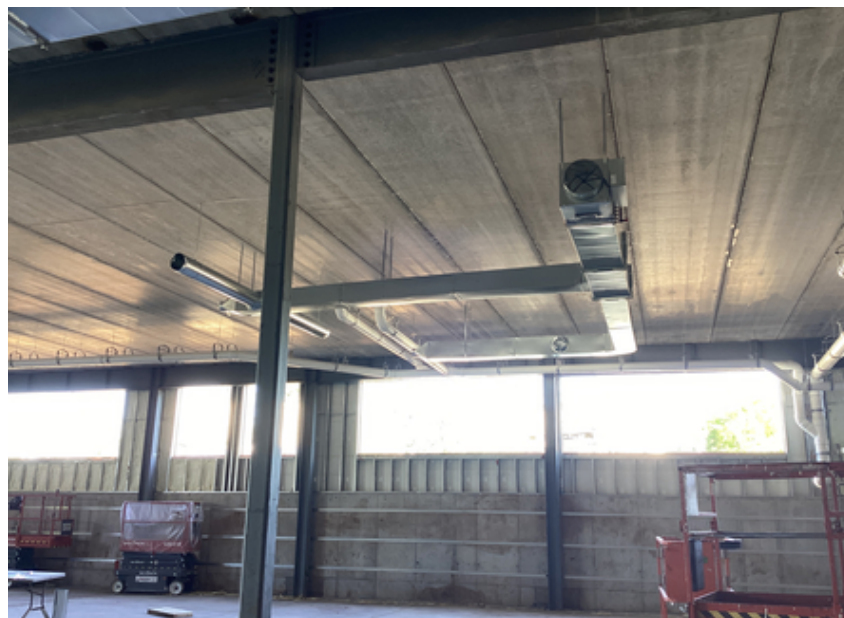
HVAC rough in Area B Music Suite
