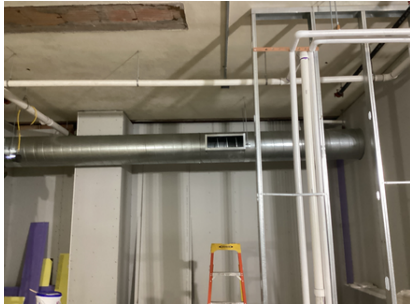
Girls' locker room mechanical rough in
