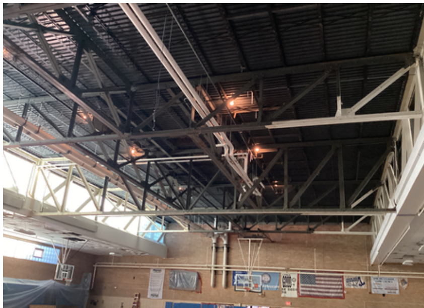
Competition gym demolition
