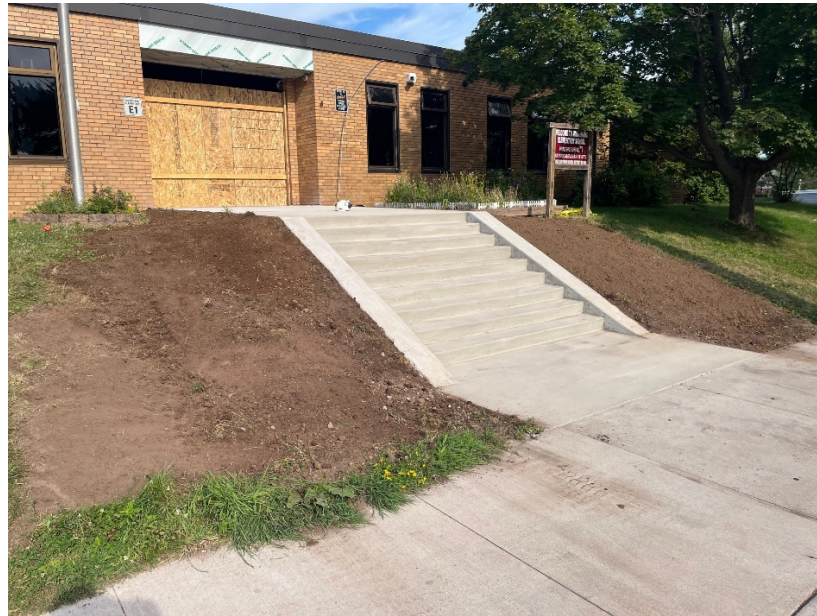
Final Grading at Perimeter of Building
