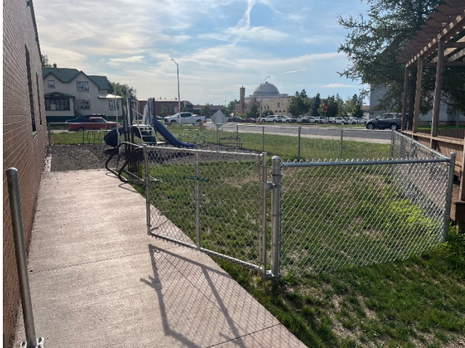
Additional Fence install
