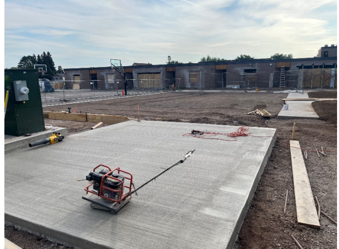
Trash Pad Concrete
