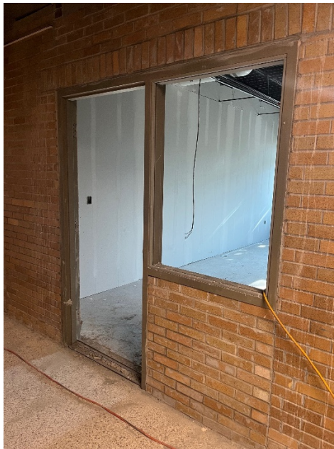
Door Cut in and Brick Patch back
