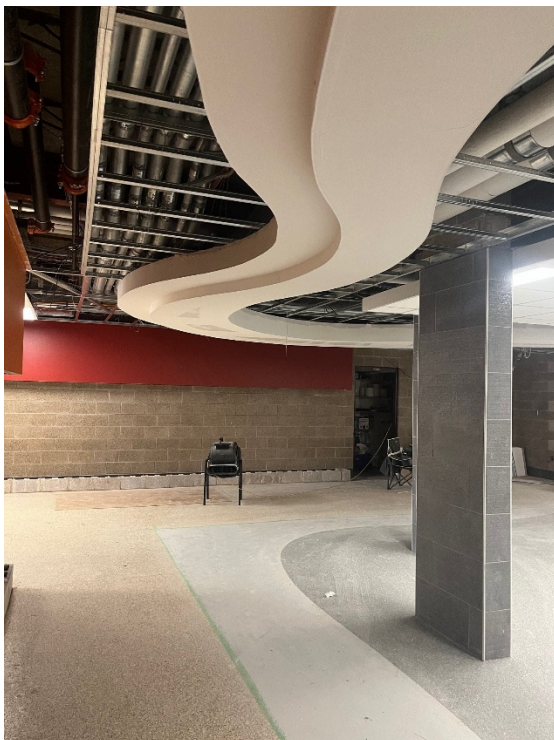
Curved Soffits in area C and Epoxy Patch back
