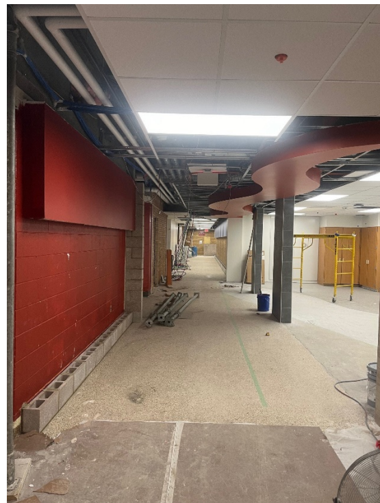
Curved Soffits in area C and Epoxy Patch back
