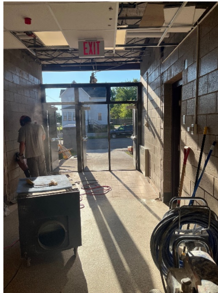
Vestibule Demolition for Replacement
