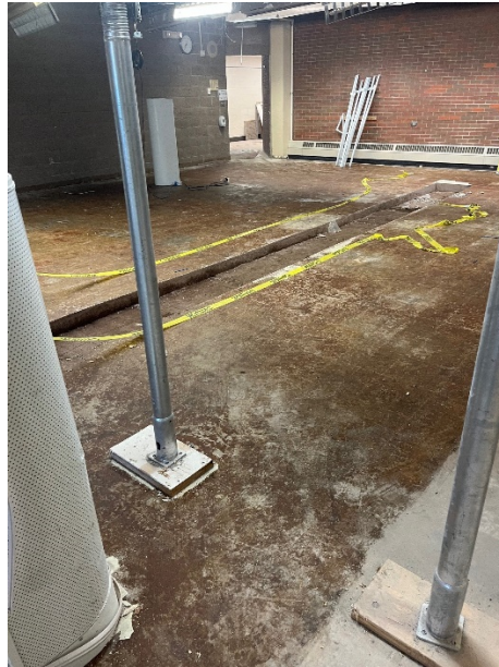
Plumbing Underground work.
