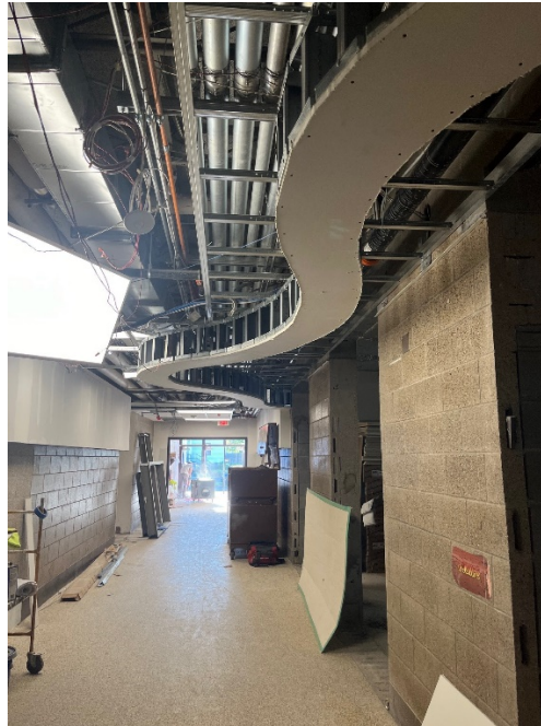
Curved Soffit Feature Framing and Drywall
