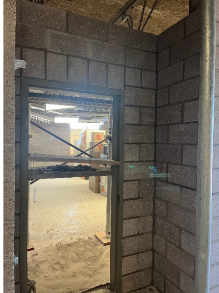
CMU Classroom Entrances
