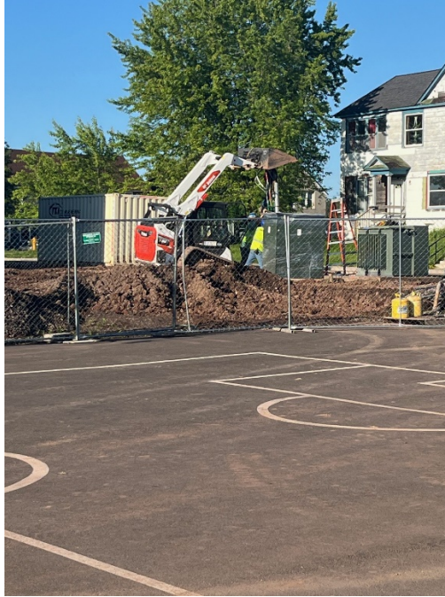
Electrical Service Prep
