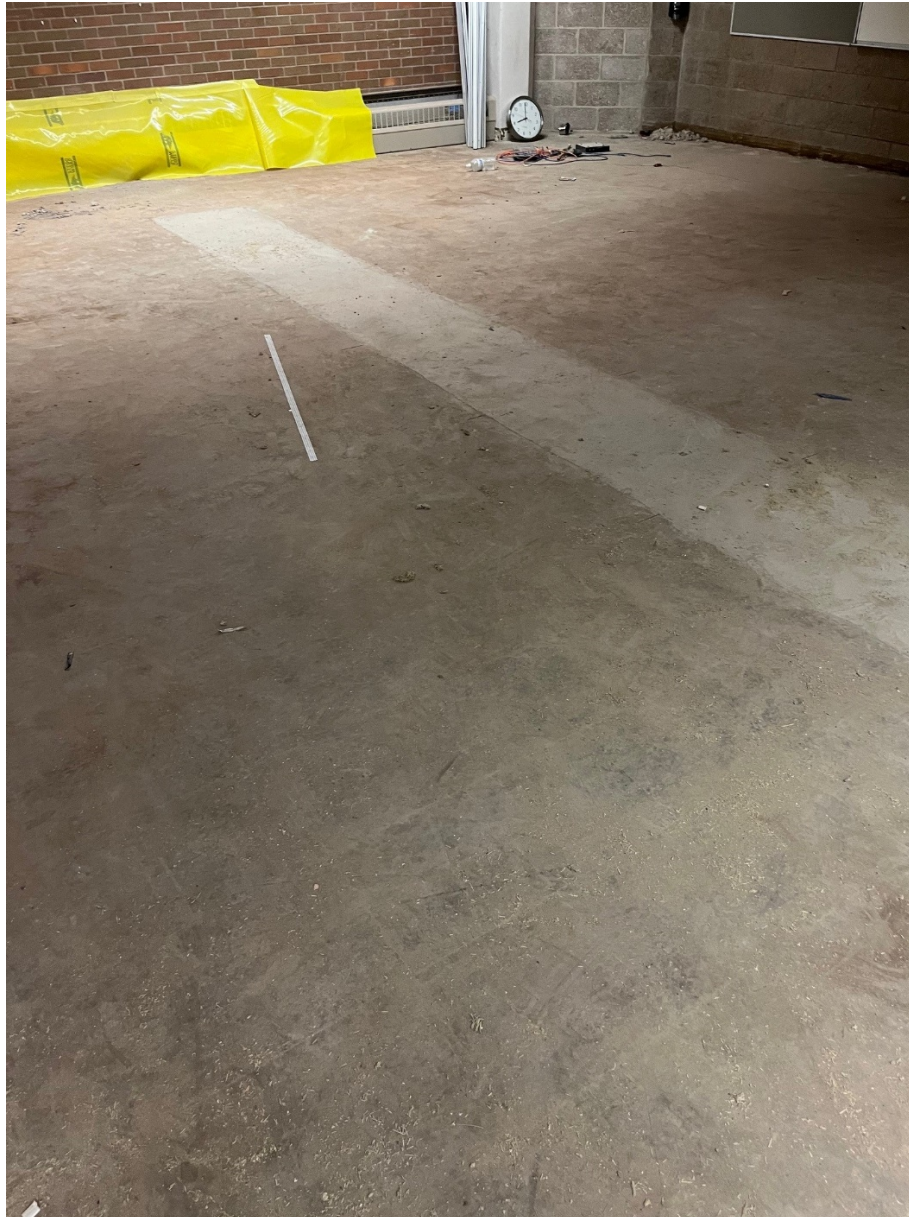
Plumbing underground Patch backs.
