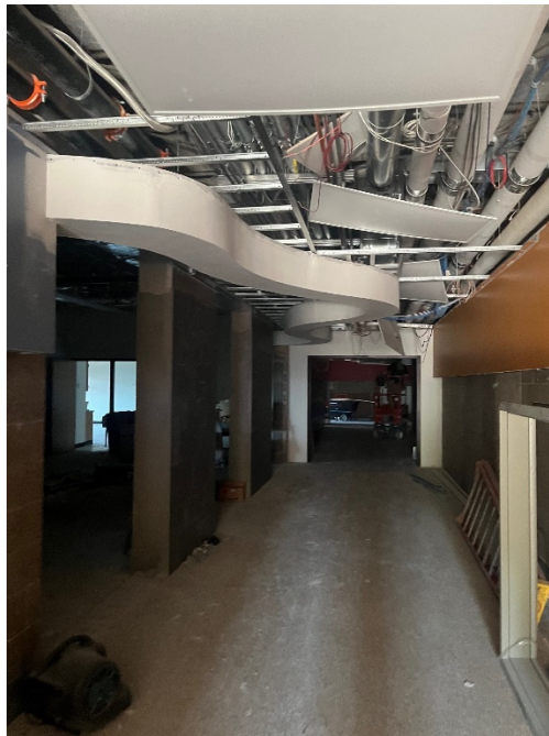
Drywall Ceiling Soffits
