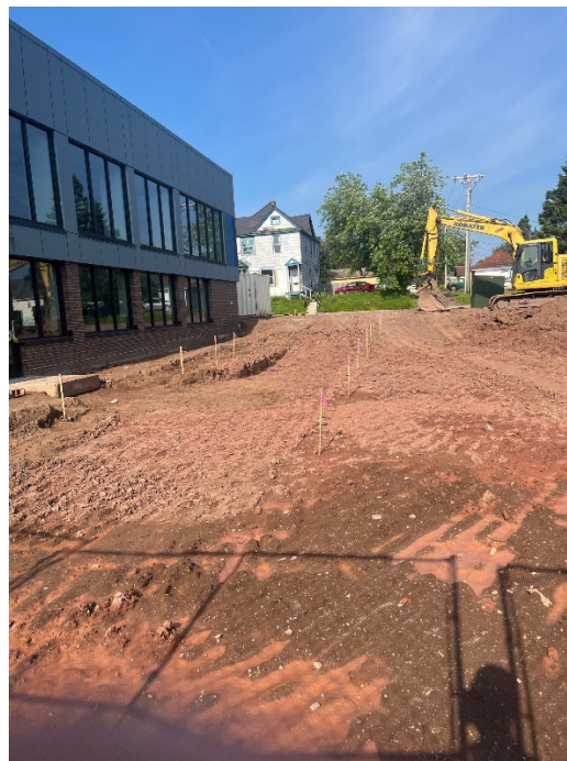
Earthwork at Sidewalk/Turf Area.
