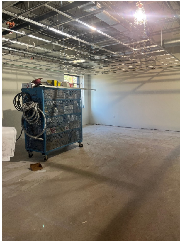
Ceiling Grid installation begins.
