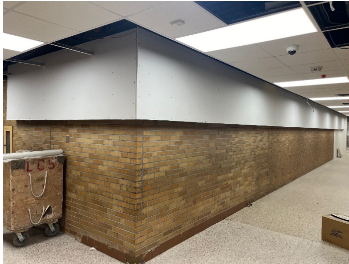
Soffit Framing
