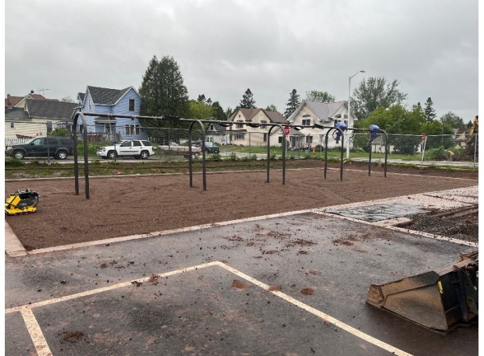
Pour-In-Place Installation (In-Progress)
