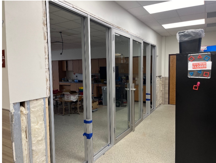
Make Space Door/Window Frame installed.
