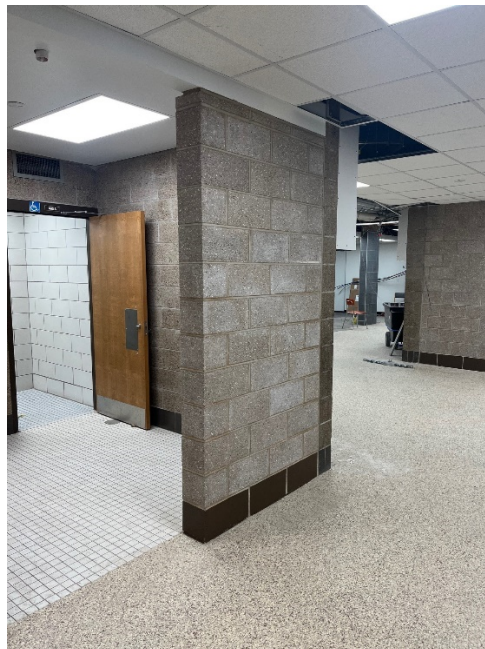
Masonry Work at Restroom in Area D.
