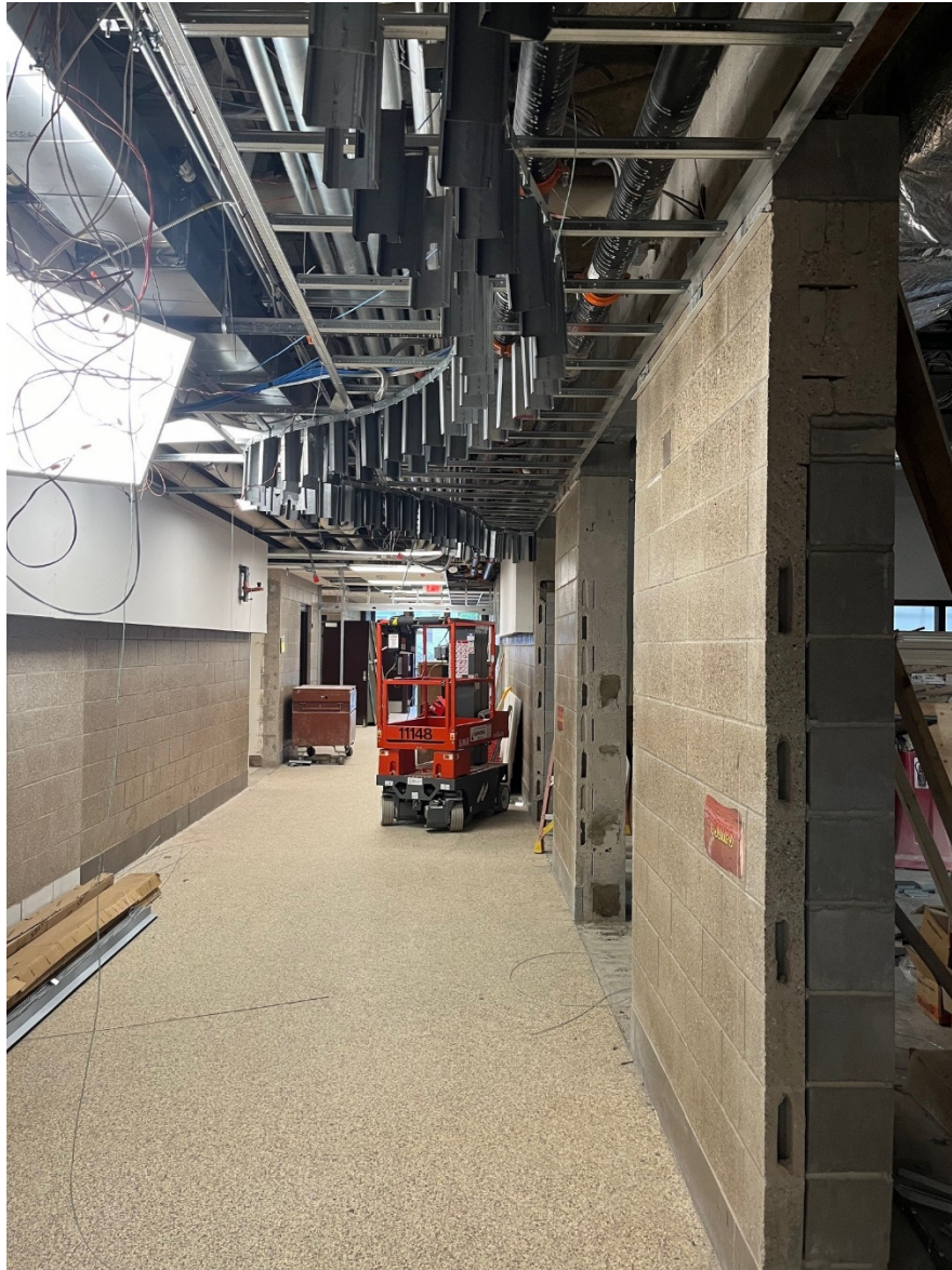
Curved Ceiling Soffit Framing
