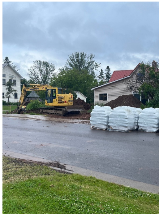
Utility Disconnects for Klinker Building Demolition.
