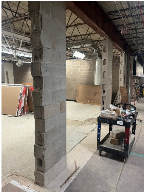
Masonry Cutting/Demolition
