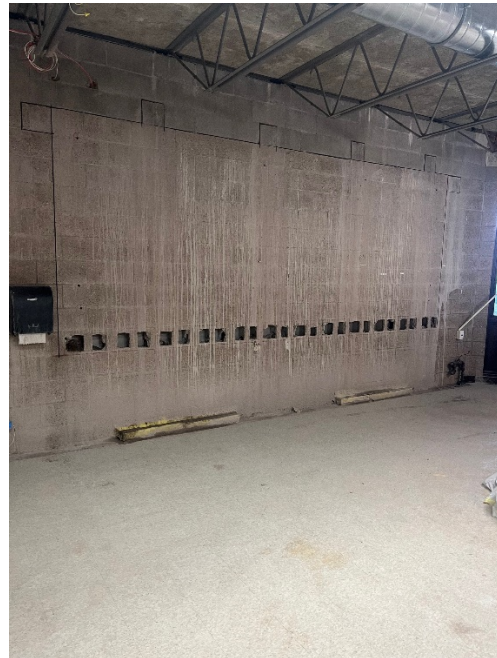
Masonry Cutting/Demolition
