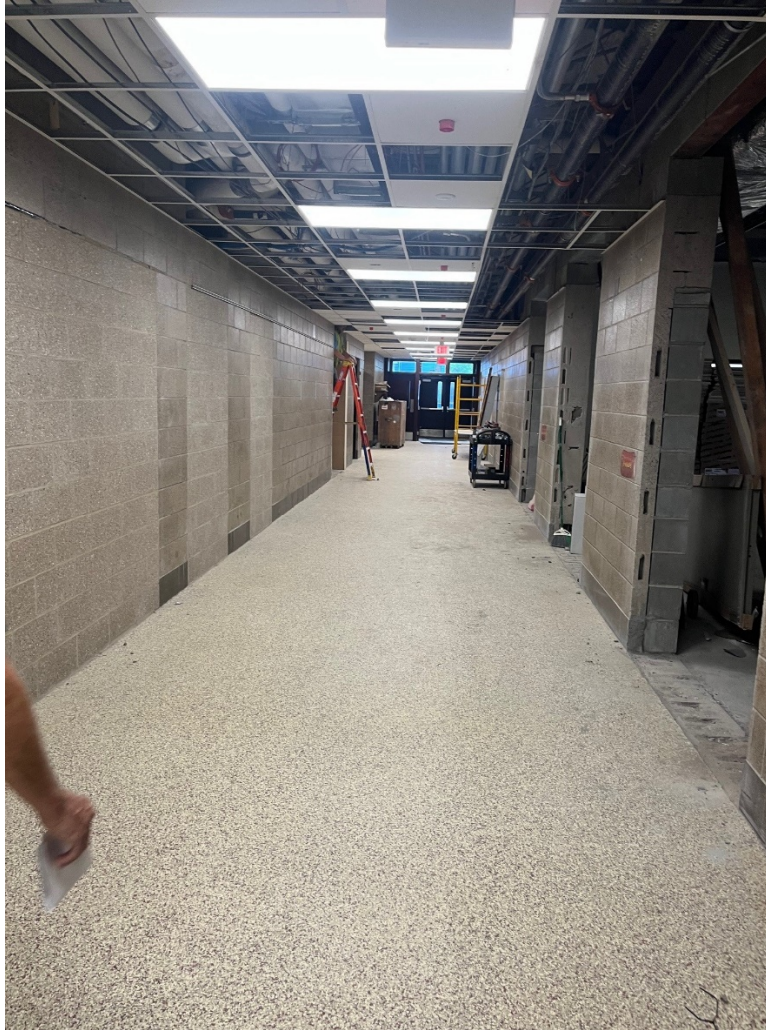
Removal of Ceiling for installation of curved soffits.
