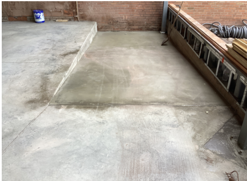
Ramp poured at Area B Music Suite
