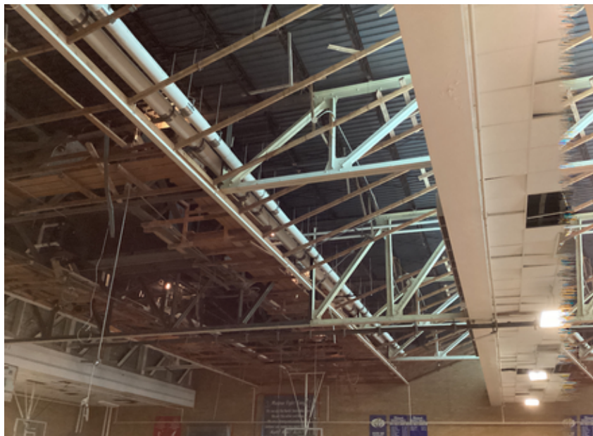
Competition gym demolition
