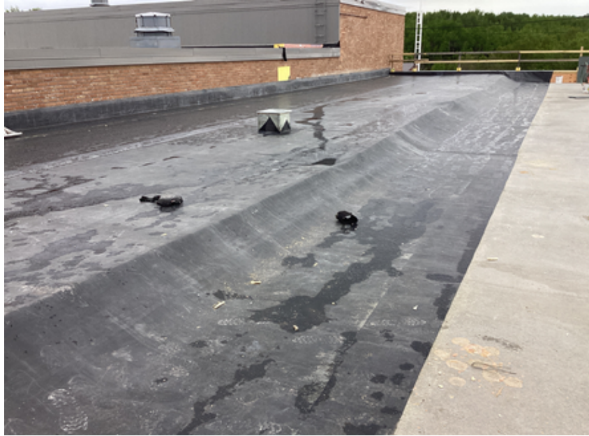
Roofing for Area B Music Suite
