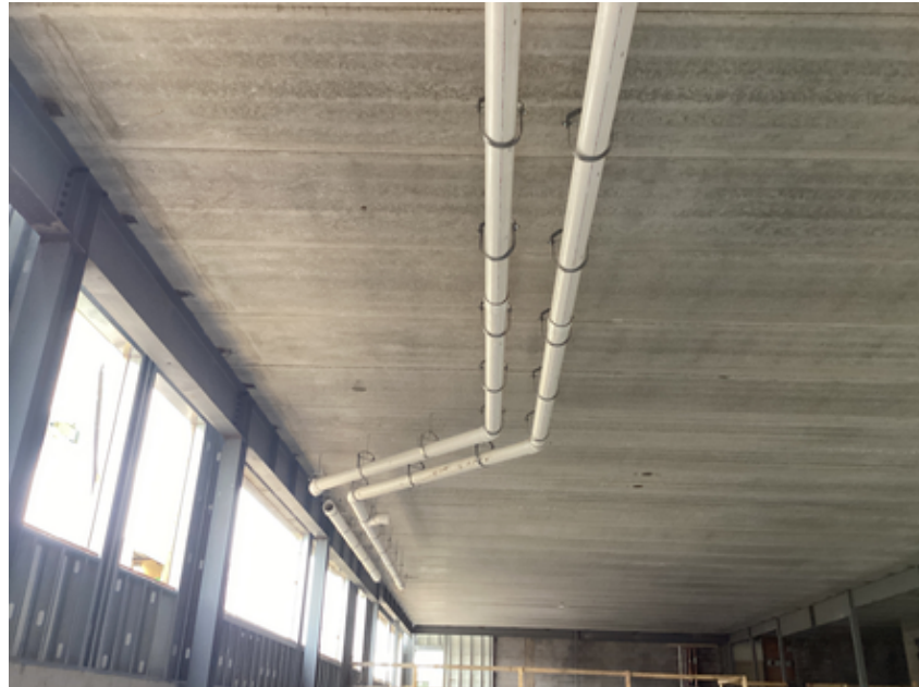
Roof drain rough in Area B Music Suite
