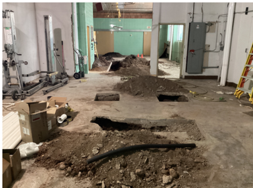
Kitchen demolition and floor removal
