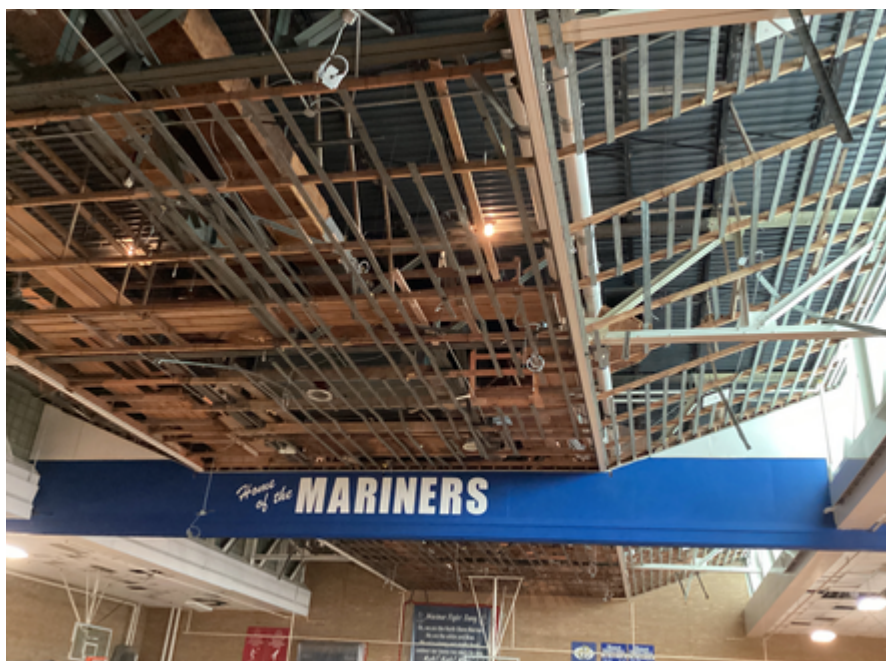
Competition gym demolition
