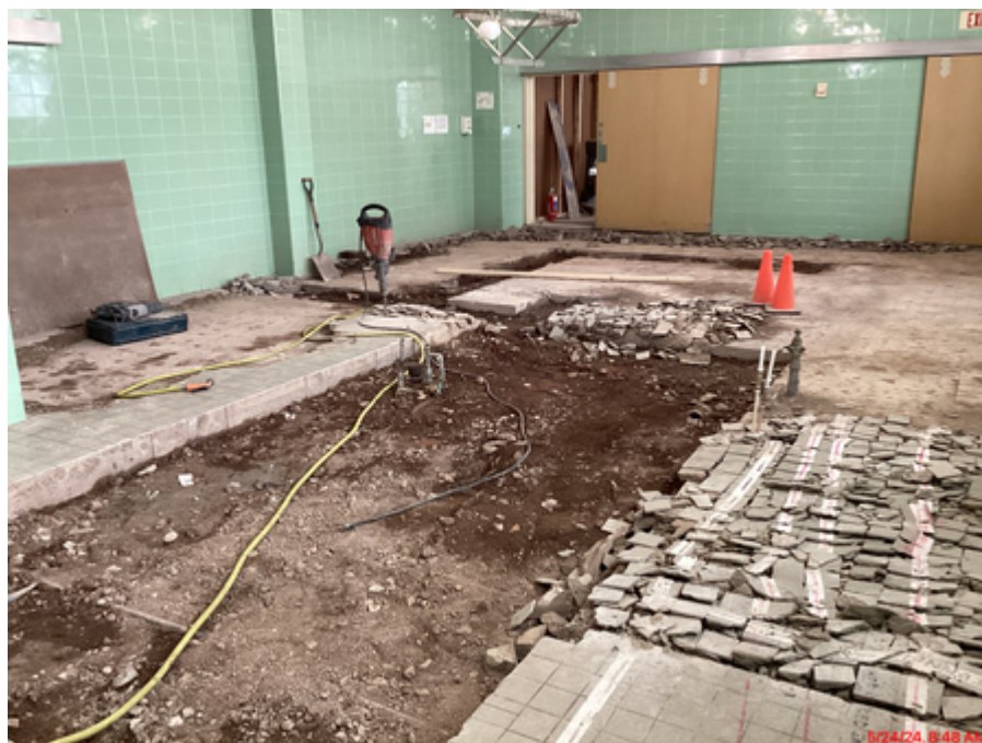
Kitchen demolition and floor removal
