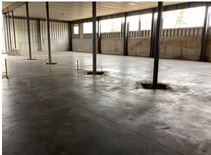
Floor poured at Area B Music Suite
