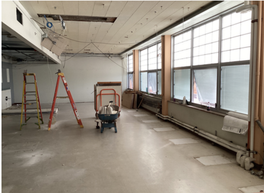
Old FACS main level Area C demolition
