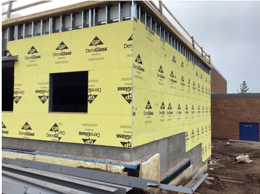
Upper level exterior wall at Area B Music Suite
