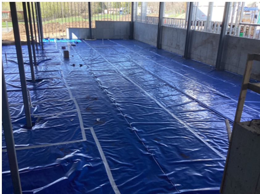
Vapor barrier installation at Area B Music Suite
