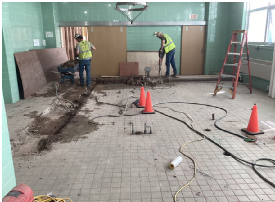
Kitchen demolition and floor removal
