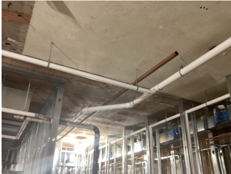
Wall framing and mechanical electrical rough in girls' locker room
