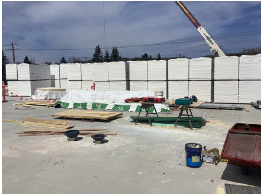
Roofing delivery and staging for Area B Music Suite
