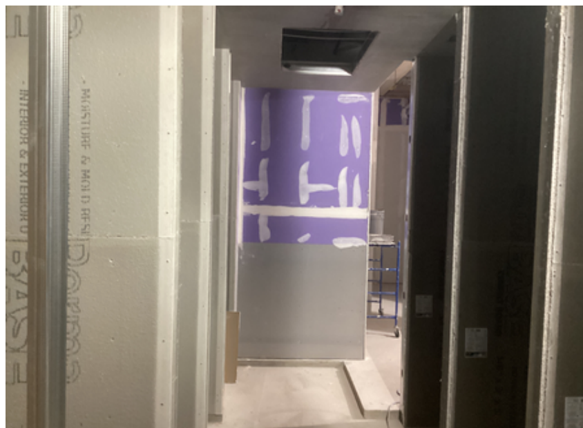
Drywall work in boys' locker room
