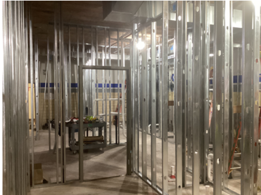
Wall framing in girls' locker room
