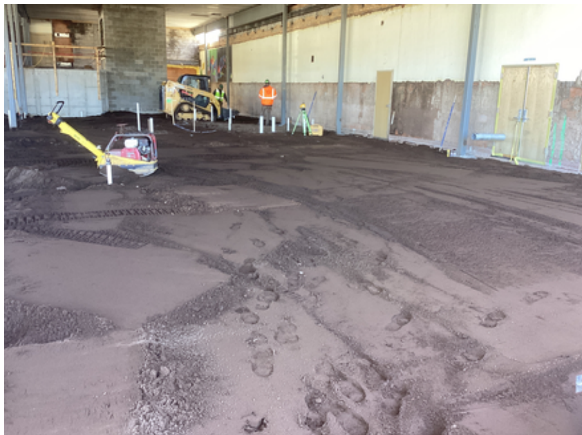
Sand cushion and prep for vapor barrier installation at Area B Music Suite
