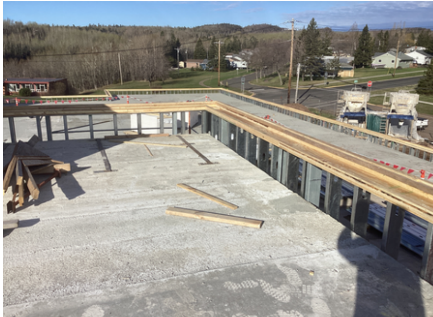
Exterior wall framing and roof blocking at Area B Music Suite
