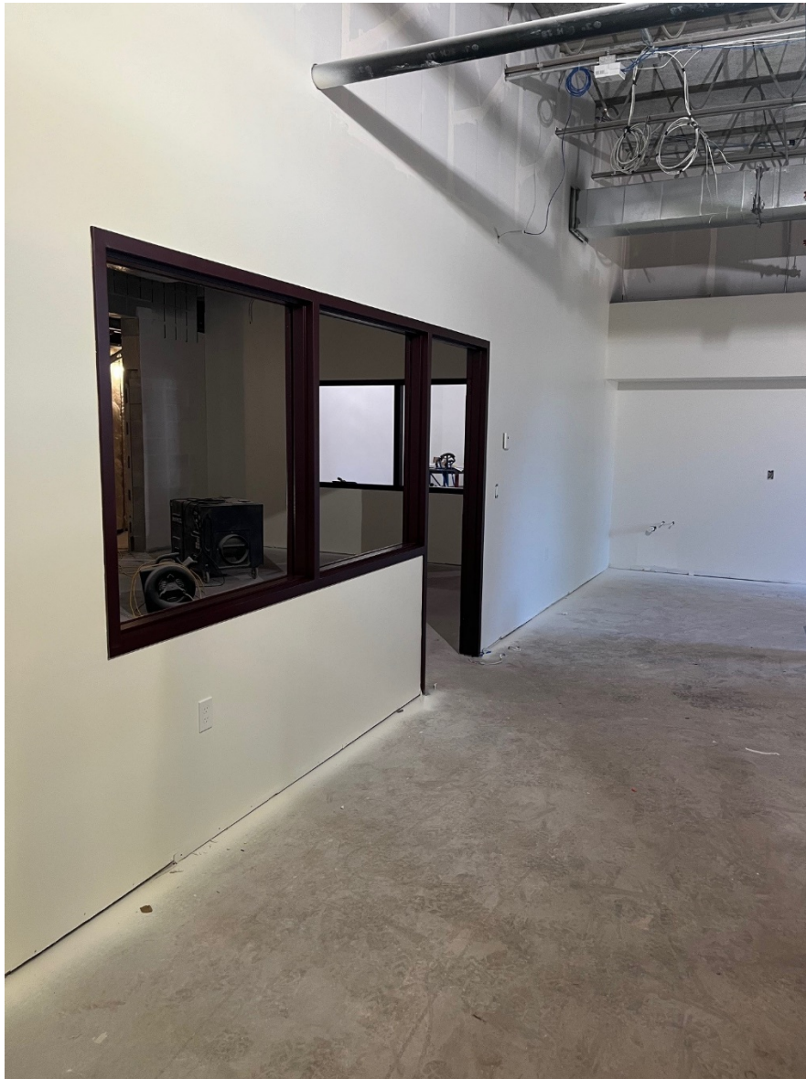
Interior room and door/window frame painting finished.
