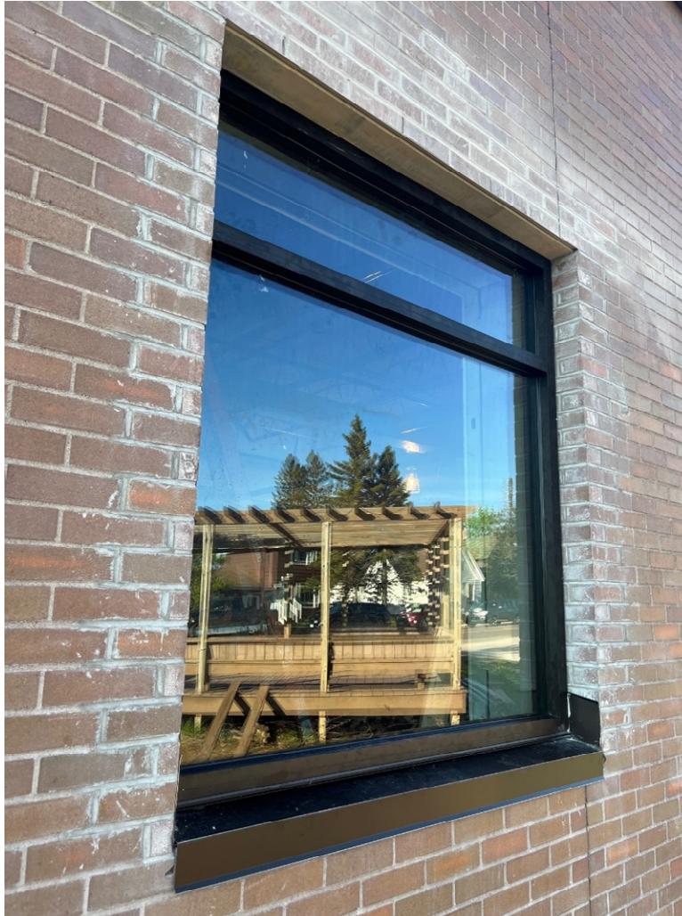
Windows installed in new Masonry Punched Openings in classrooms.
