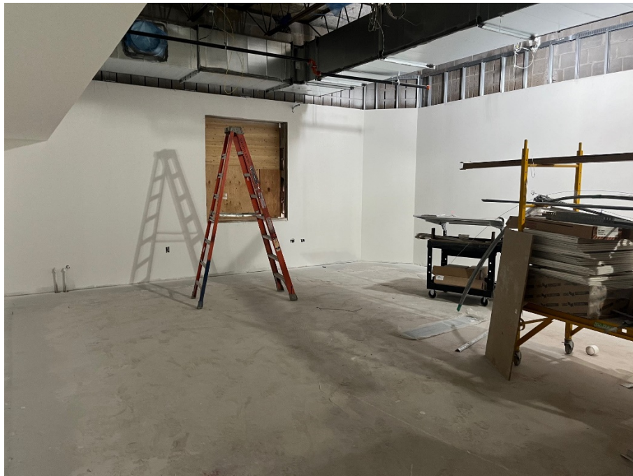
Painting of walls at Kindergarten Suite
