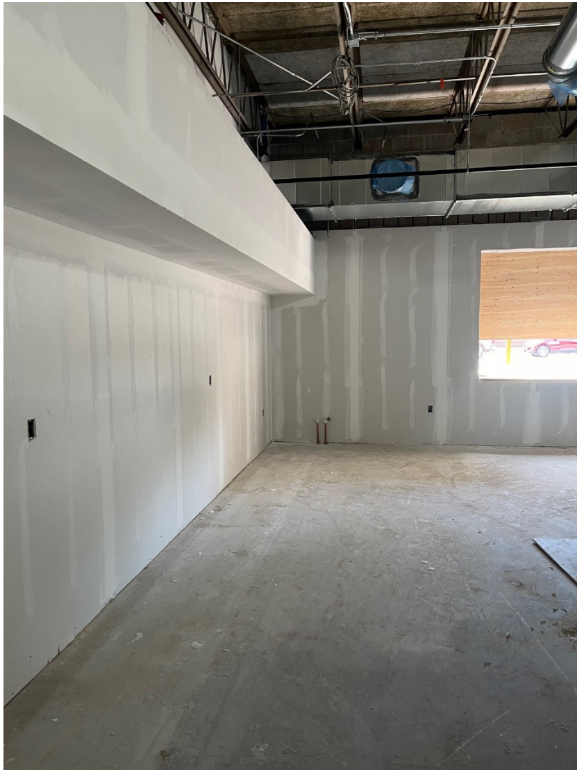
Soffiting Framed and taped.
